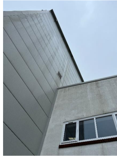
Photograph 10 - Picture taken facing the western side of Unit 14 highlighting good condition of joints amongst Unit 14 building and bindings as well as underside of guttering.
