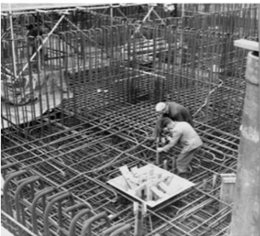
Workmen constructing formwork for the machine base in the kiln building at the Solway Chemical Works in Whitehaven
