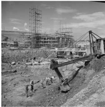
Construction of the Solway Chemical Works in Whitehaven, showing excavation in progress for the kiln building with limestone being cleared and tested for faults
