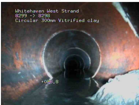
8299X_b6d85f02-8f59-4d60-9979-0fab5b24b70a_20210127_135420_484.jpg, 00:07:00, 39.00 m Connection defective at 2 o'clock, diameter: 100mm,
