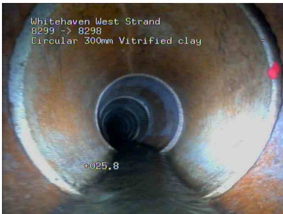
8299X_c4c59bfa-c898-4e95-ad7a-4c7b2ab741fb_20210127_134752_746.jpg, 00:04:45, 25.00 m Crack, longitudinal at 12 o'clock
