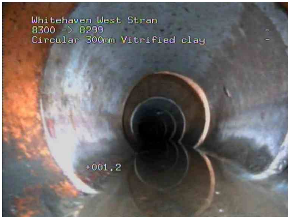
8300X_3c2c67f0-8708-4fc2-80d0-f0ac6a738835_20210127_0 85230_436.jpg, 00:00:30, 1.20 m Open joint, medium, start
