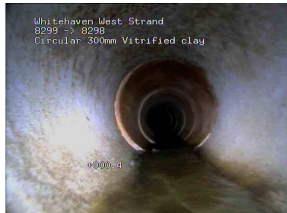
8299X_c65224e6-83d1-4db8-af87-a4a6a3af1c21_20210127_133833_441.jpg, 00:00:45, 38.80 m Joint displaced, medium, finish
