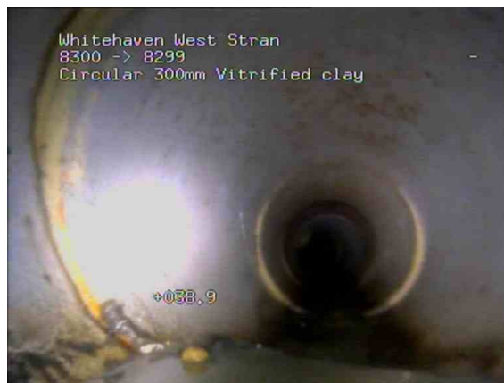
8300X_027885fd-0194-4e7f-bac6-b044ea709bdc_20210127_091553_409.jpg, 00:09:29, 39.00 m Open joint, medium, finish
