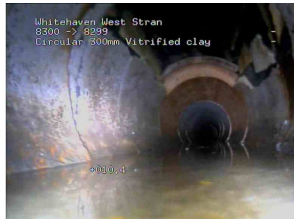
8300X_f105f827-fbda-4d9e-92ed-00a32f8fc4f0_20210127_09 0258_468.jpg, 00:03:26, 10.40 m Broken pipe from 11 o'clock to 1 o'clock, Old access point -
