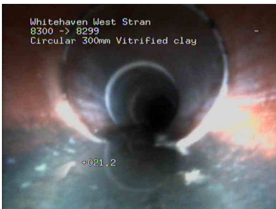
8300X_32a619e3-77b9-40d4-b051-c5e59971465d_20210127 _090741_536.jpg, 00:05:59, 21.20 m Crack, longitudinal at 10 o'clock, cracked along length
