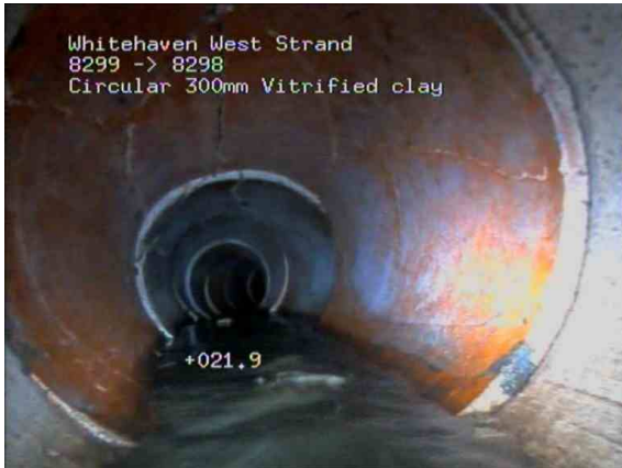
8299X_c0c2e085-19d3-4d35-9365-69e53ab72fa0_20210127_134558_593.jpg, 00:04:07, 21.90 m Cracks, multiple from 8 o'clock to 3 o'clock
