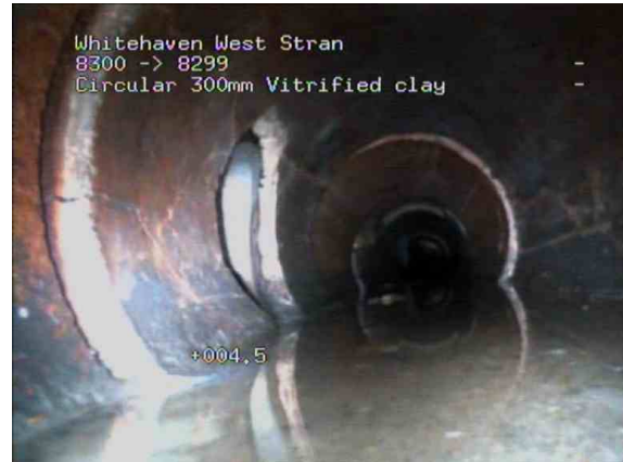
8300X_b3112f4e-bf19-41eb-9e4f-7ef07e9f85ff_20210127_085 419_027.jpg, 00:01:33, 3.40 m Open joint, medium, finish
