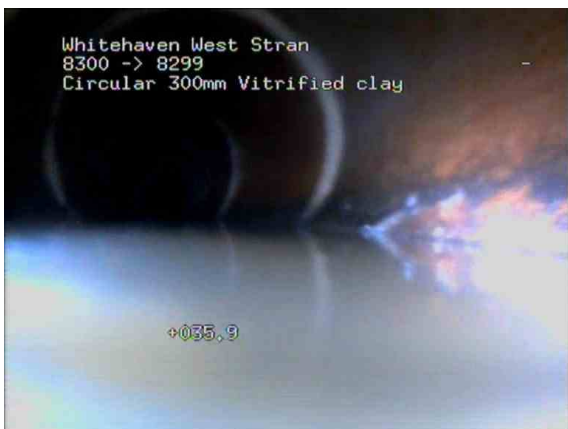
8300X_48e006d8-774a-473d-af09-569ac07c0270_20210127_091344_834.jpg, 00:08:53, 35.00 m Turbid water level, 15% of the vertical dimension
