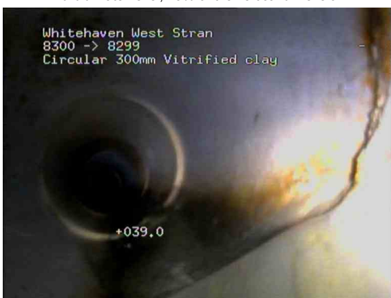
8300X_ae598982-02d1-4213-b522-96764395a7cc_20210127_091719_289.jpg, 00:09:48, 39.00 m Survey abandoned, Drop in drain
