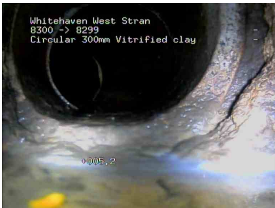
8300X_9122fc2a-8fcb-4f3d-87fb-abdfed0b38db_20210127_08 5659_944.jpg, 00:02:15, 5.20 m Connection defective at 9 o'clock, diameter: 100mm, defunct
