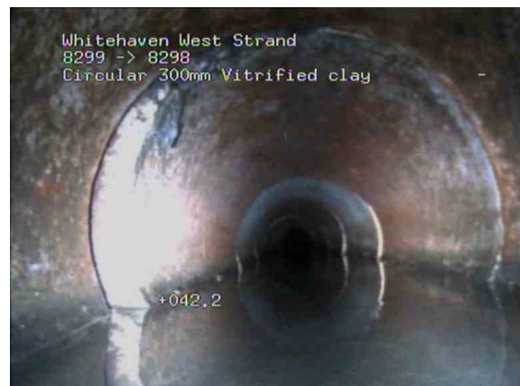
8299X_9b51a8fc-0a0b-4498-b374-753f6b89415c_20210127_135551_203.jpg, 00:07:53, 42.20 m Turbid water level, 20% of the vertical dimension
