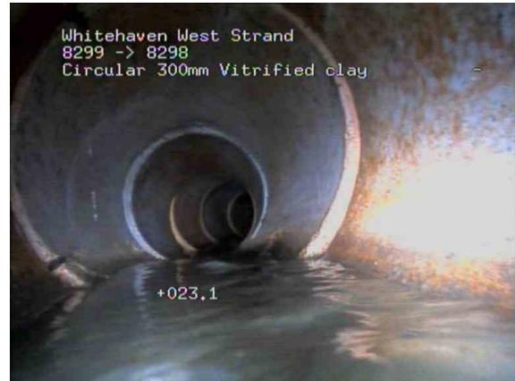
8299X_83244a2d-91ac-4d1f-8f90-816056fd9270_20210127_134650_463.jpg, 00:04:18, 23.10 m Crack, longitudinal at joint at 7 o'clock
