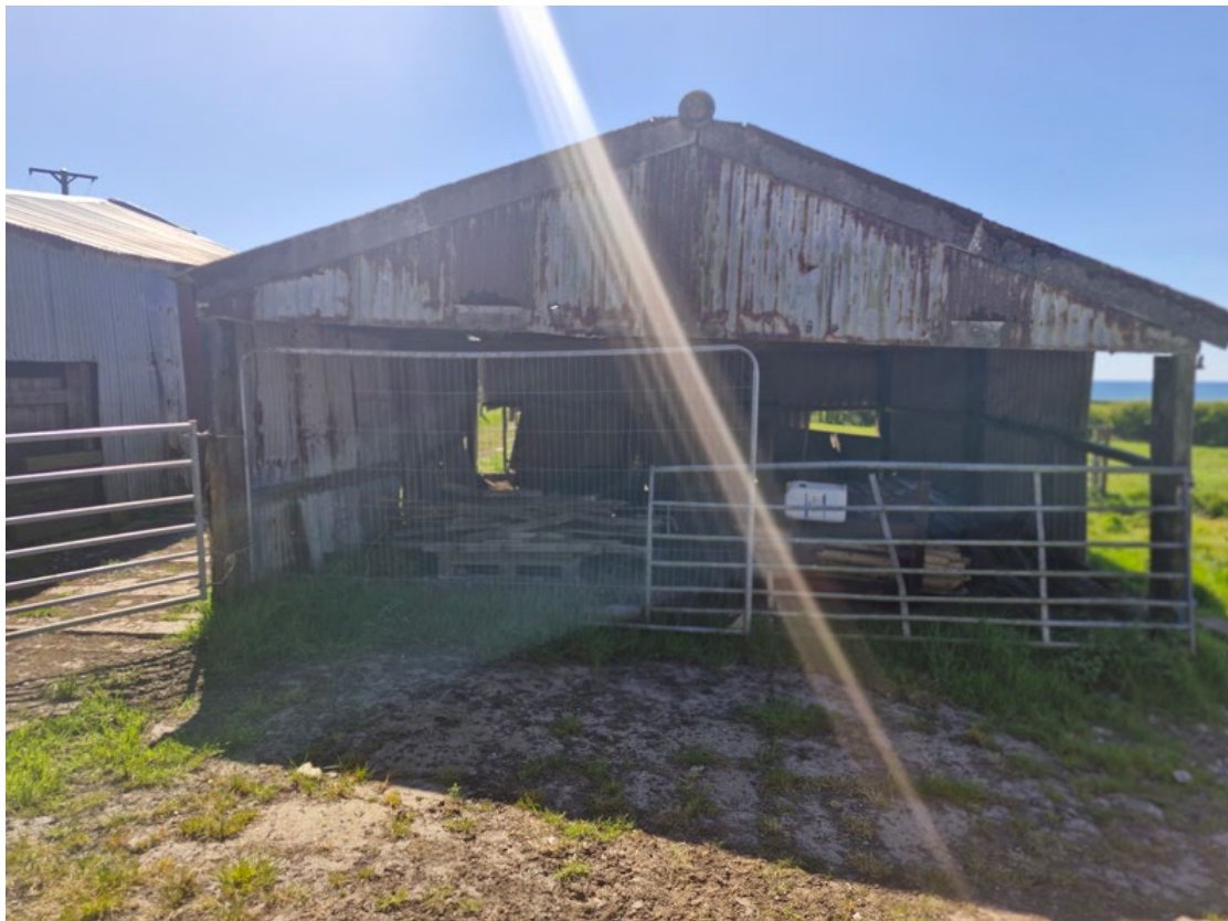
PHOTO 06 DETACHED TIMBER PORTAL SHED
