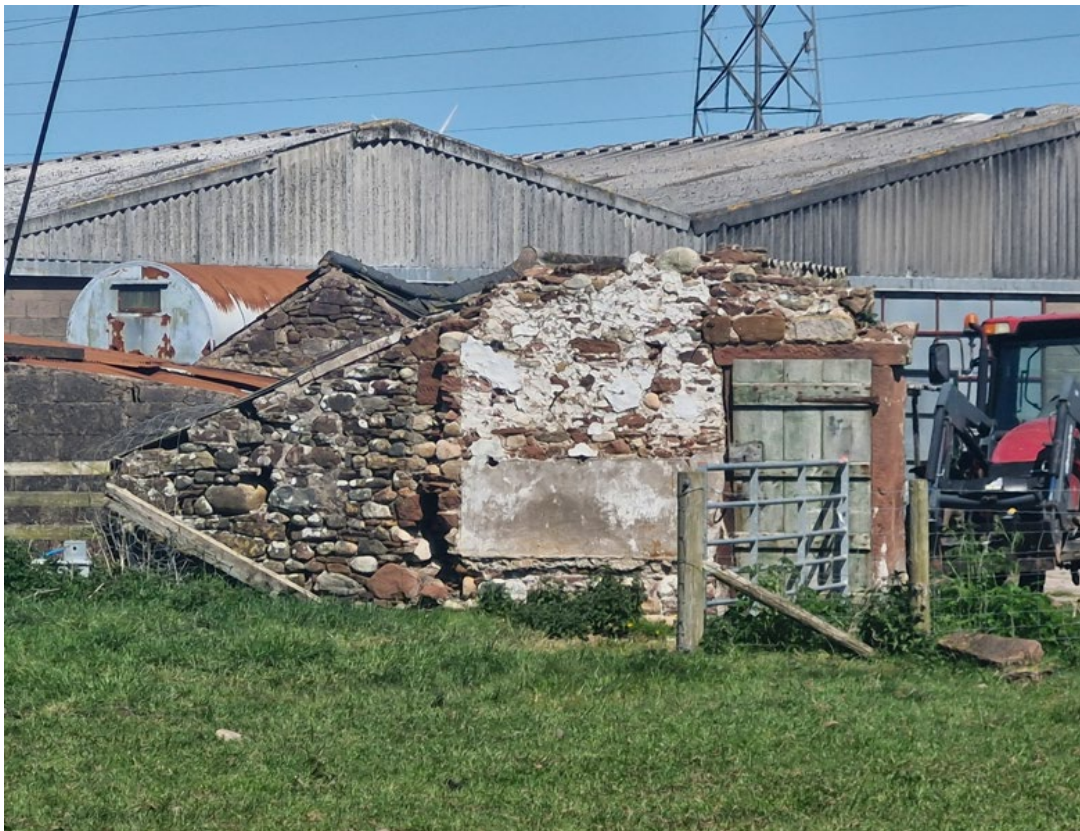
PHOTO 04 VIEW LEFT HAND MASONRY BUILDINGS
