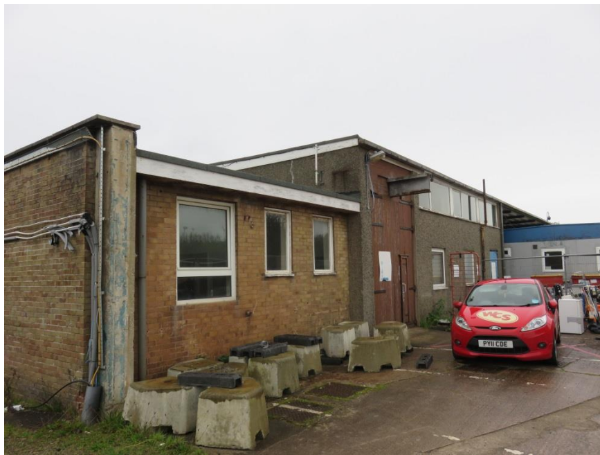
Photograph 10: Building W1 – south-east of building, exterior of workshop area.
