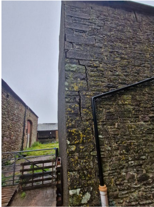
PHOTO 01 SIDE VIEW ON GABLE AND CRACKING
