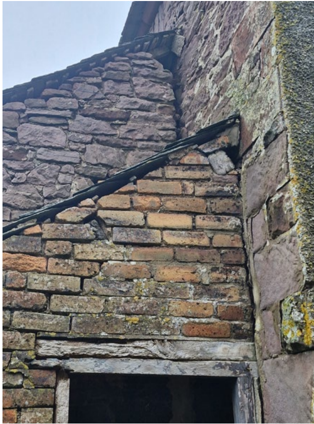
PHOTO 03 REAR LEAN TO SEPARATION CACKS
