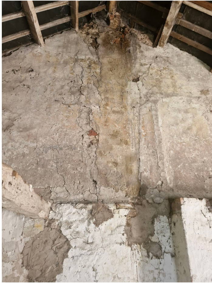
PHOTO 03 VIEW ON BARN INTERNAL PARTY WALL WITH HOUSE
