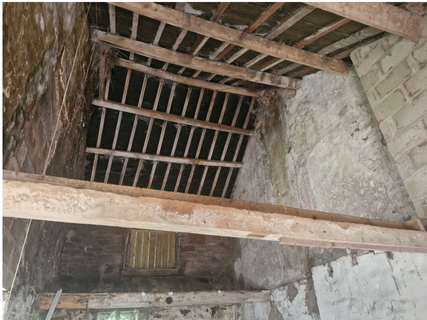
PHOTO 04 TYPICAL VIEW ON ROOF STRUCTURE AND FLOOR BEAM
