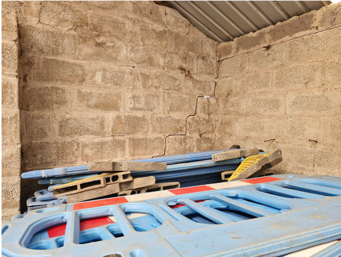
PHOTO 09 CRACKING TO REAR WALL BARN 4
