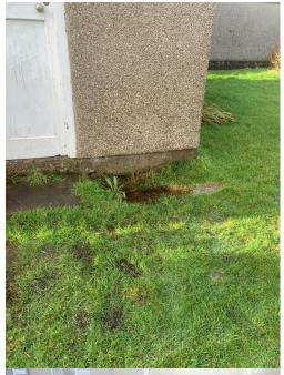
As can be seen in the attached pictures, flooding is an issue in this area of the garden. Presently the drain from the garage roof just goes into the ground and saturates the surrounding grass.
