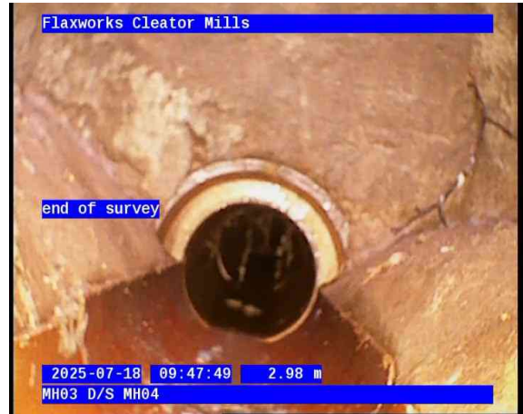
MH03-MH04-18-07-2025-008.jpg, 00:00:27, 2.98 m Finish node, manhole, reference: MH04
