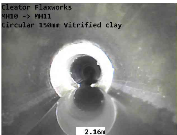
MH10-MH11-02-10-2025-020.jpg, 00:00:36, 2.16 m Pipe material changes to vitrified clay at this point
