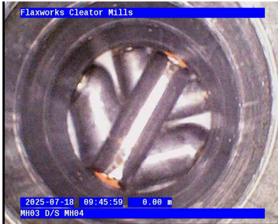
MH03-MH04-18-07-2025-007.png, 00:00:00, 0.00 m Start node, manhole, reference: MH03
