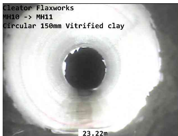
MH10-MH11-02-10-2025-025.jpg, 00:04:10, 23.22 m Pipe material changes to epoxy at this point, patch liner
