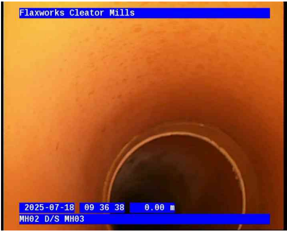
MH02-MH03-18-07-2025-005.jpg, 00:00:00, 0.00 m Start node, manhole, reference: MH02
