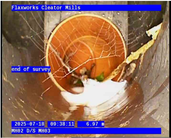
MH02-MH03-18-07-2025-006.jpg, 00:01:32, 6.97 m Finish node, manhole, reference: MH03, end of survey
