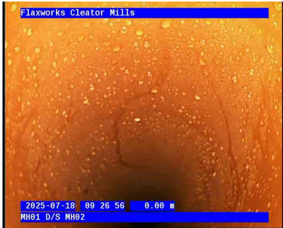
MH01-MH02-18-07-2025-003.jpg, 00:00:00, 0.00 m Start node, manhole, reference: MH01
