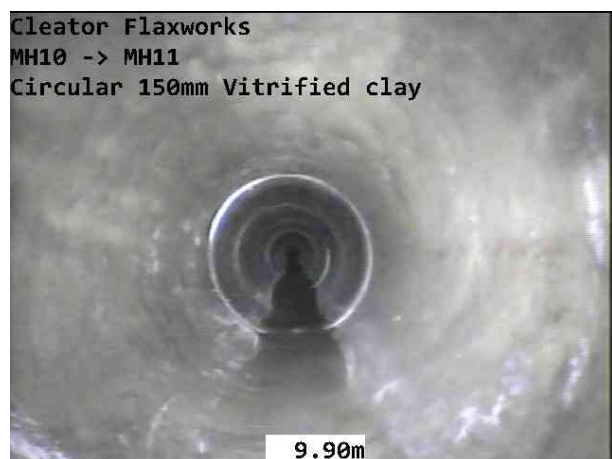
MH10-MH11-02-10-2025-024.jpg, 00:01:57, 9.90 m Pipe material changes to vitrified clay at this point
