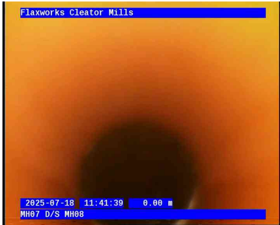
MH07-MH08-02-10-2025-011.jpg, 00:00:00, 0.00 m Start node, manhole, reference: MH07
