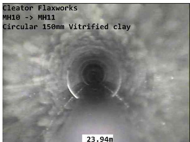
MH10-MH11-02-10-2025-026.jpg, 00:04:17, 23.94 m Pipe material changes to vitrified clay at this point
