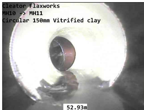
MH10-MH11-02-10-2025-029.jpg, 00:09:47, 52.93 m Pipe material changes to epoxy at this point, patch liner
