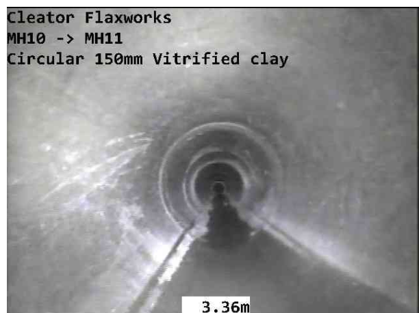
MH10-MH11-02-10-2025-022.jpg, 00:00:48, 3.38 m Pipe material changes to vitrified clay at this point
