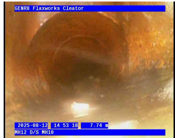
MH12-MH10-13-08-2025-016.jpg, 00:00:43, 7.74 m Junction at 3 o'clock, 150mm dia
