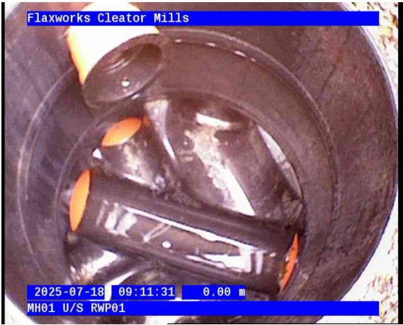
MH01-RWP01-18-07-2025-001.png, 00:00:00, 0.00 m Start node, manhole, reference: MH01
