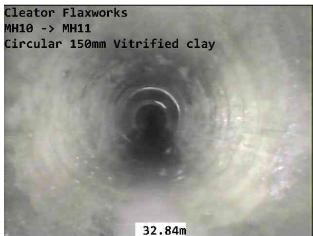
MH10-MH11-02-10-2025-028.jpg, 00:05:53, 32.84 m Pipe material changes to vitrified clay at this point
