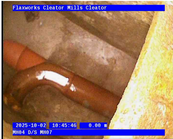
MH04-MH07-02-10-2025-009.png, 00:00:00, 0.00 m Start node, manhole, reference: MH04
