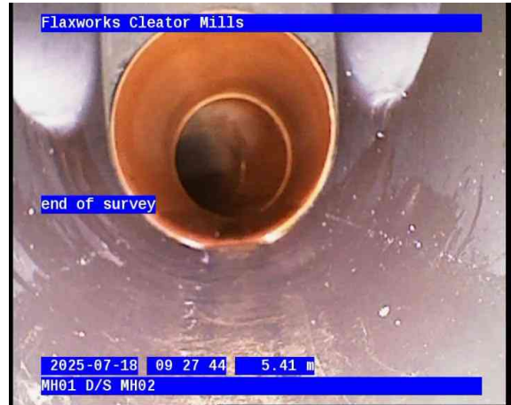
MH01-MH02-18-07-2025-004.jpg, 00:00:48, 5.41 m Finish node, manhole, reference: MH02, end of survey
