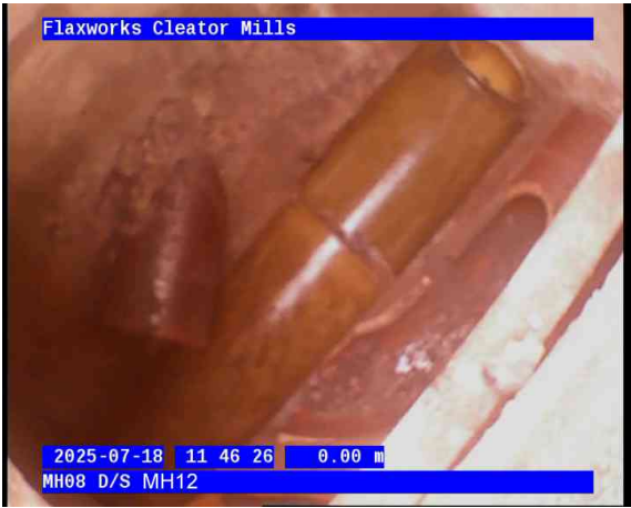
MH08-MH12-21-08-2025-013.png, 00:00:00, 0.00 m Start node, manhole, reference: MH08
