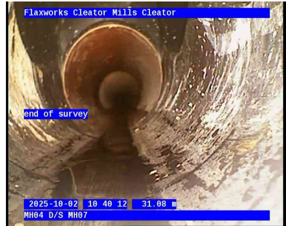
MH04-MH07-02-10-2025-010.jpg, 00:02:00, 31.08 m Finish node, manhole, reference: MH07, end of survey
