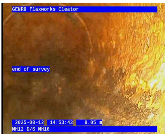
MH12-MH10-13-08-2025-017.jpg, 00:00:58, 8.05 m Finish node, manhole, reference: MH10, end of survey
