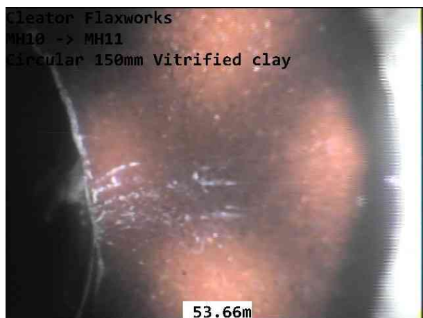
MH10-MH11-02-10-2025-030.jpg, 00:09:58, 53.66 m Pipe material changes to vitrified clay at this point
