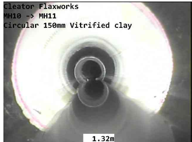
MH10-MH11-02-10-2025-019.jpg, 00:00:29, 1.32 m Pipe material changes to epoxy at this point, patch liner
