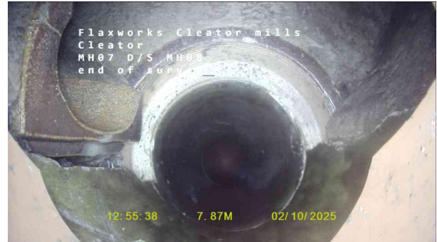
MH07-MH08-02-10-2025-012.jpg, 00:01:34, 7.87 m Finish node, manhole, reference: MH08, end of survey
