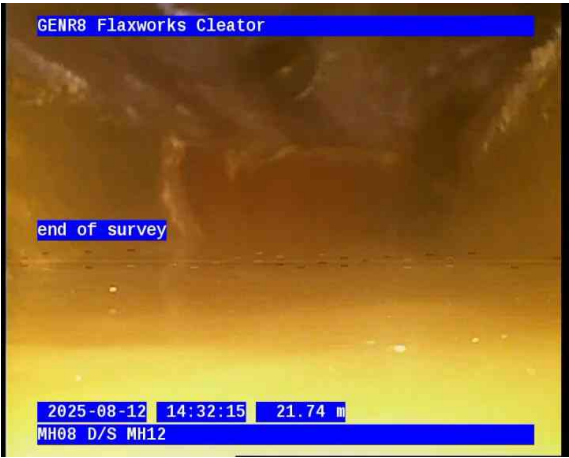
MH08-MH12-21-08-2025-014.jpg, 00:06:53, 21.74 m Finish node, manhole, reference: MH12, end of survey
