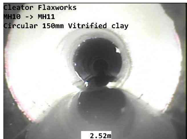
MH10-MH11-02-10-2025-021.jpg, 00:00:40, 2.52 m Pipe material changes to epoxy at this point, patch liner
