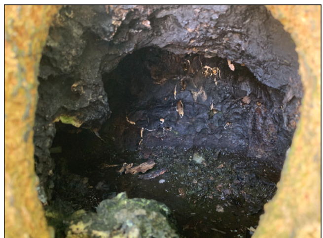
Figure 4 - Extensive cavity and decayed wood
