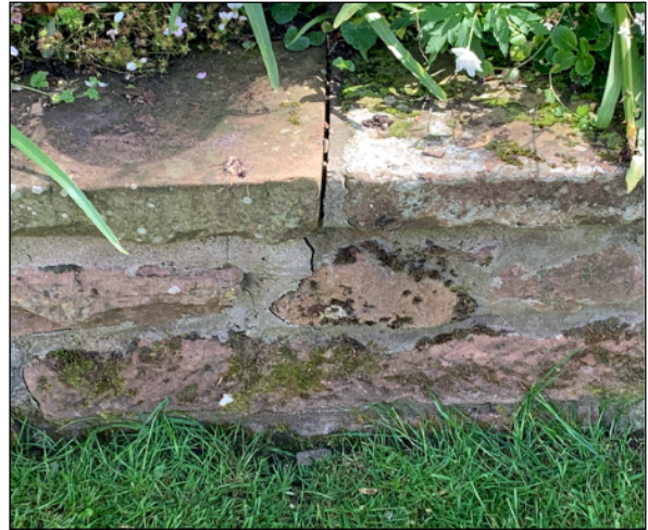
Figure 11 - Crack in retaining bed wall
