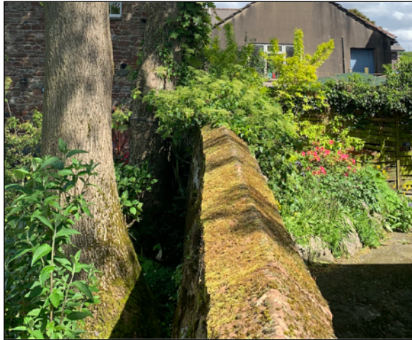
Figure 10 - Ash and proximity to boundary wall causing movement
