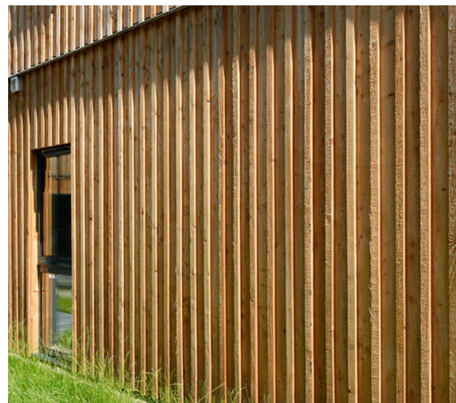
Larch cladding – board on board
