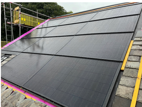
Solar panels during construction
