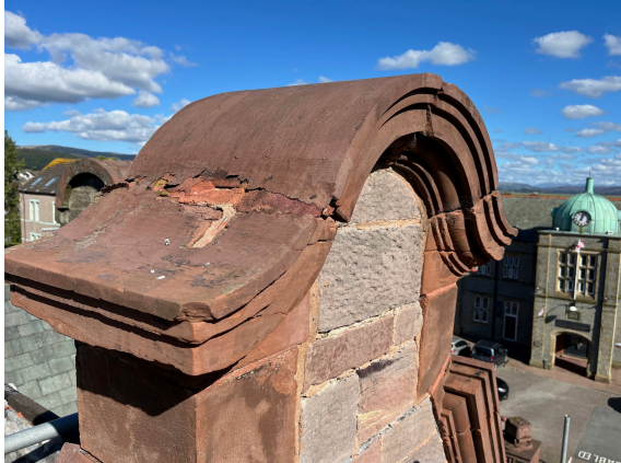
Existing stone parapet
