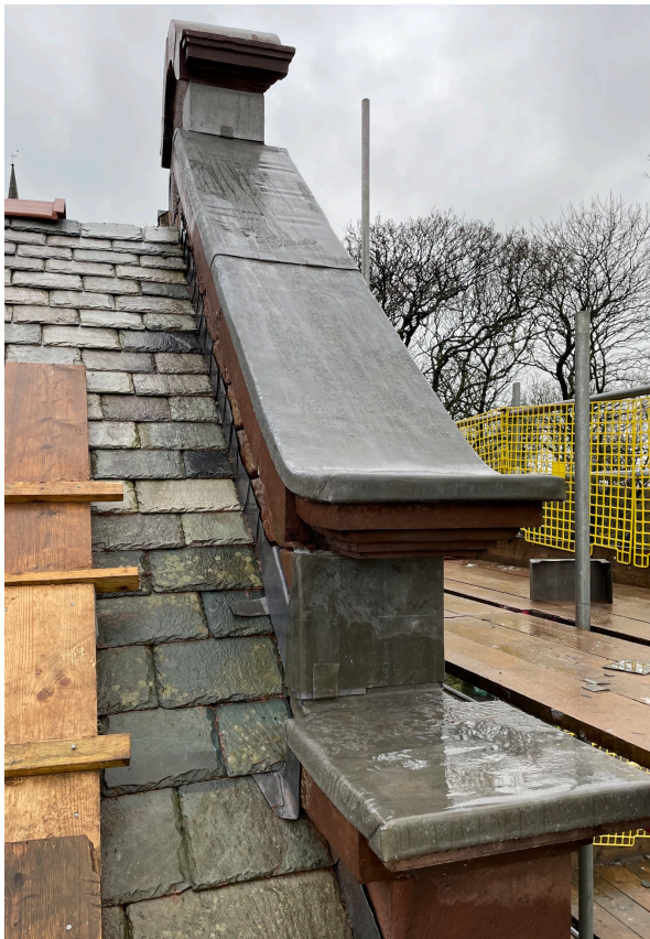
Lead cappings installed
