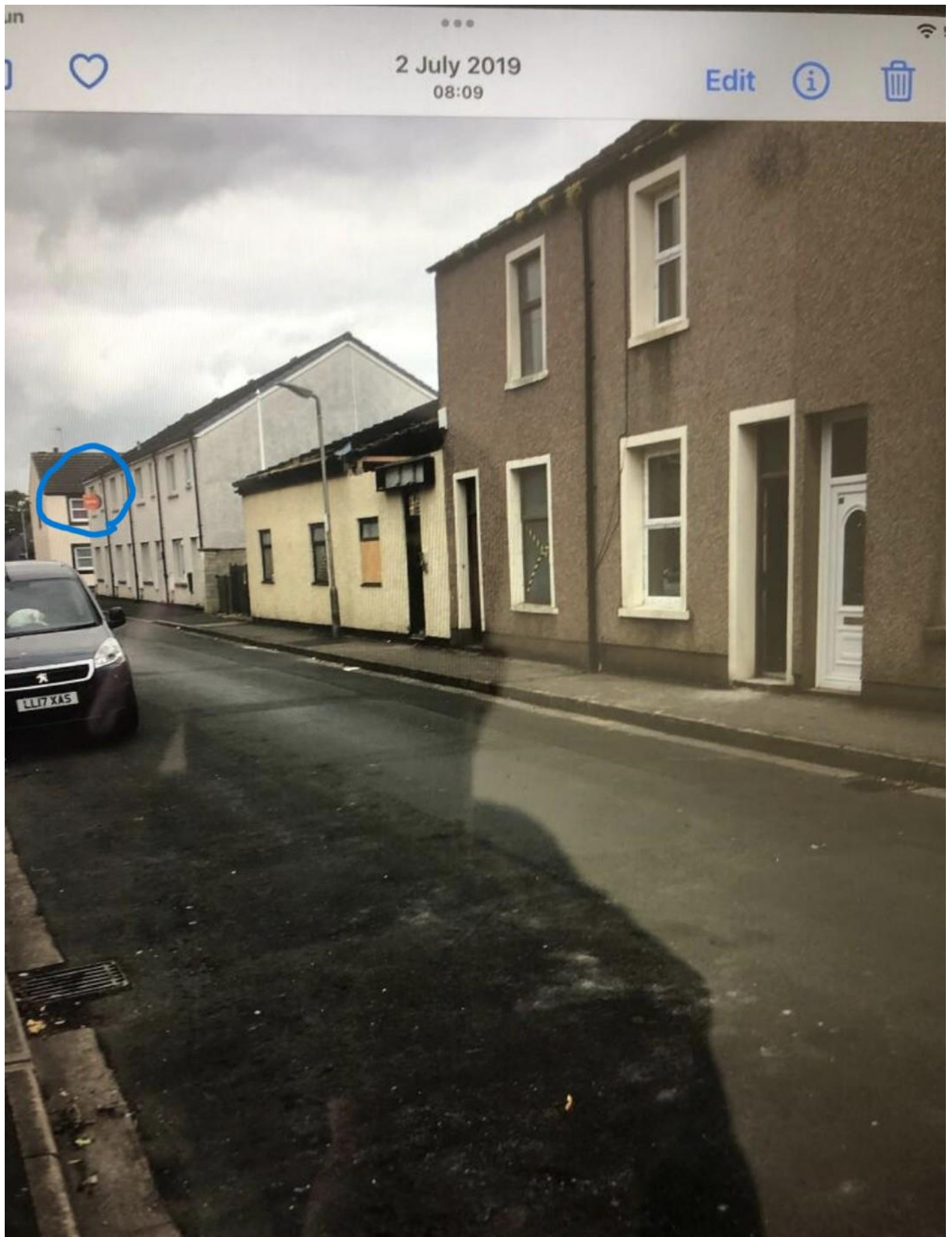
Part demolished and Corrie sale sign – 2019
