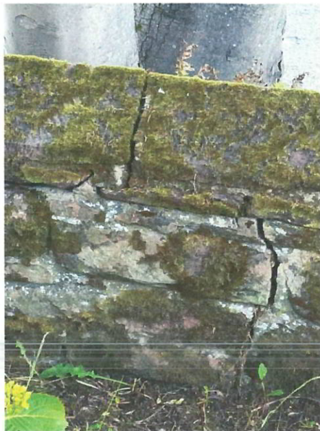
Trees 5 & 6 are outside the garden wall but are still on our property. They lean out and overhang onto St Bees Main Street and Seacroft Drive. They are also causing damage to the garden wall.
