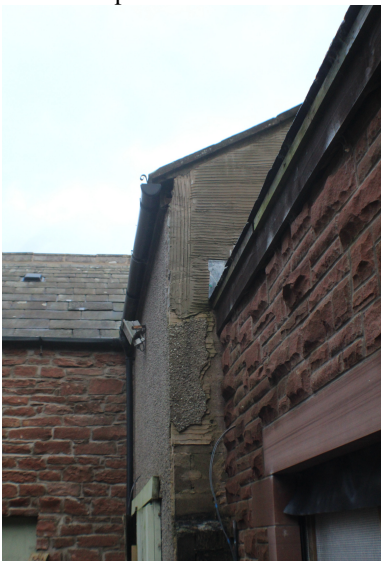
View of potential west fascia access
