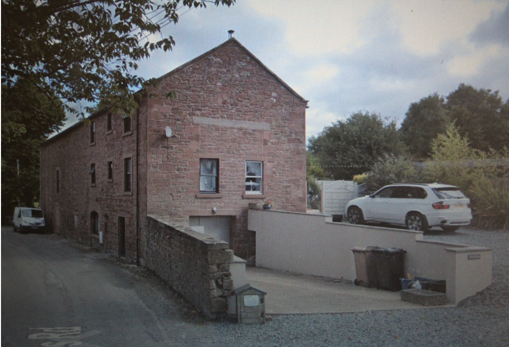
Barn viewed from the southwest
