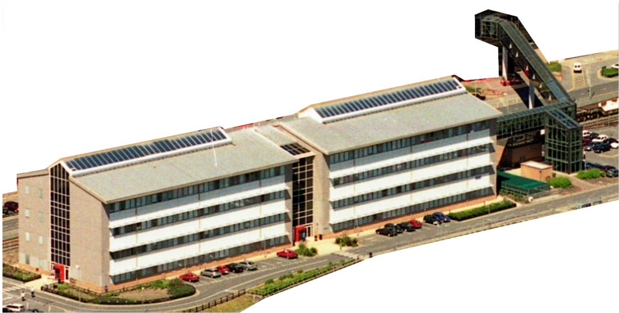
THORP Management Centre (TMC) in 1999 with the complete link bridge in place at the north end
