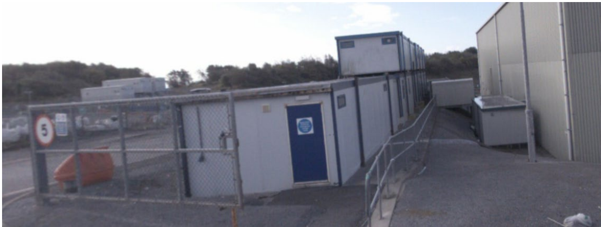
Figure 1: North end of the MRFOC site showing the single stacked Portacabin in the foreground with double stacked ones behind, the Glasdon hut on the right at the far end of the safety railing and the small walkway extension Portacabin next to the wall of the MRF.
