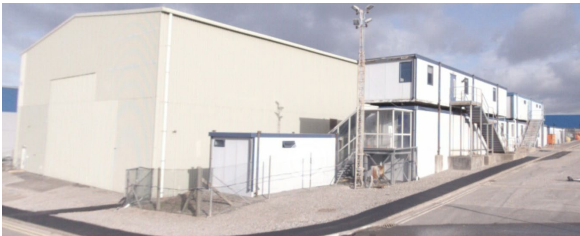
Figure 2: Southeastern elevation of the MRFOC showing the access steps to the top Portacabins, the covered walkway and single storey Portacabin at the south end.
