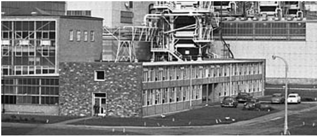
Figure 2 – The Calder Hall Administration Building taken from the south in 1959, showing the rock clad end gable wall and the new windows of the single storey workshop on the west side
