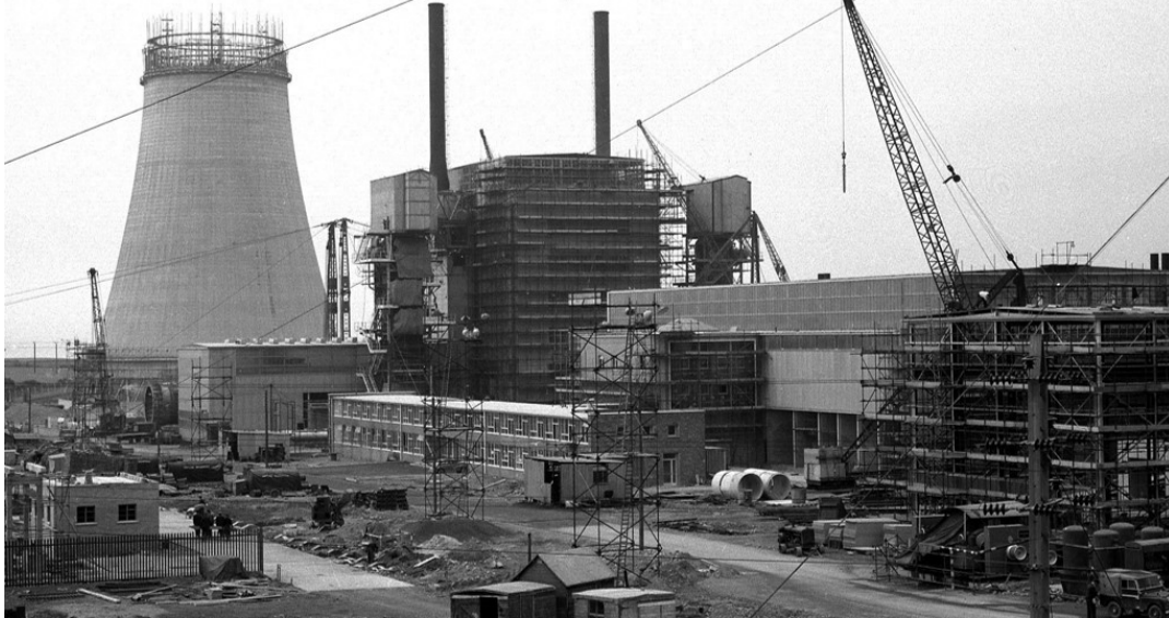
Figure 1 – Calder Hall Administration Building during construction taken in 1955
