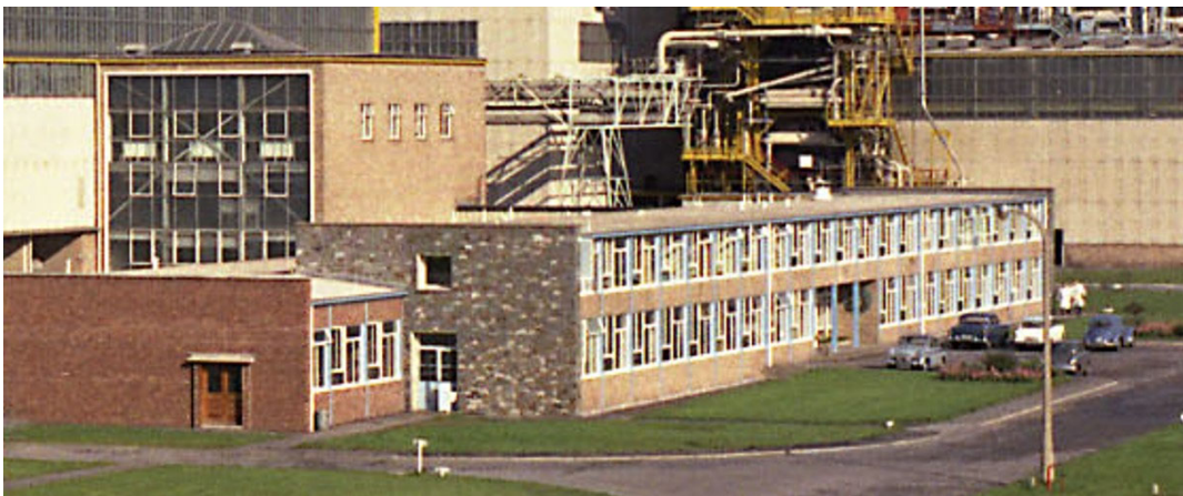
Figure 3 – The CHAB in 1962 taken from the south end showing the extension to the workshop
