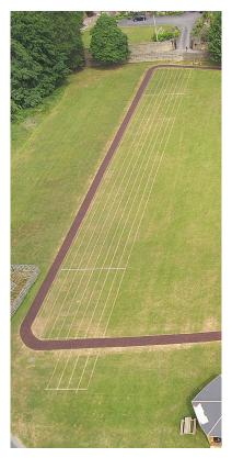
Once installed and fully cured the surface is considered inert and nontoxic. The surfacing uses large quantities of recycled tyres, one of the most intractable wastes known to man and therefore has excellent environmental credentials.
