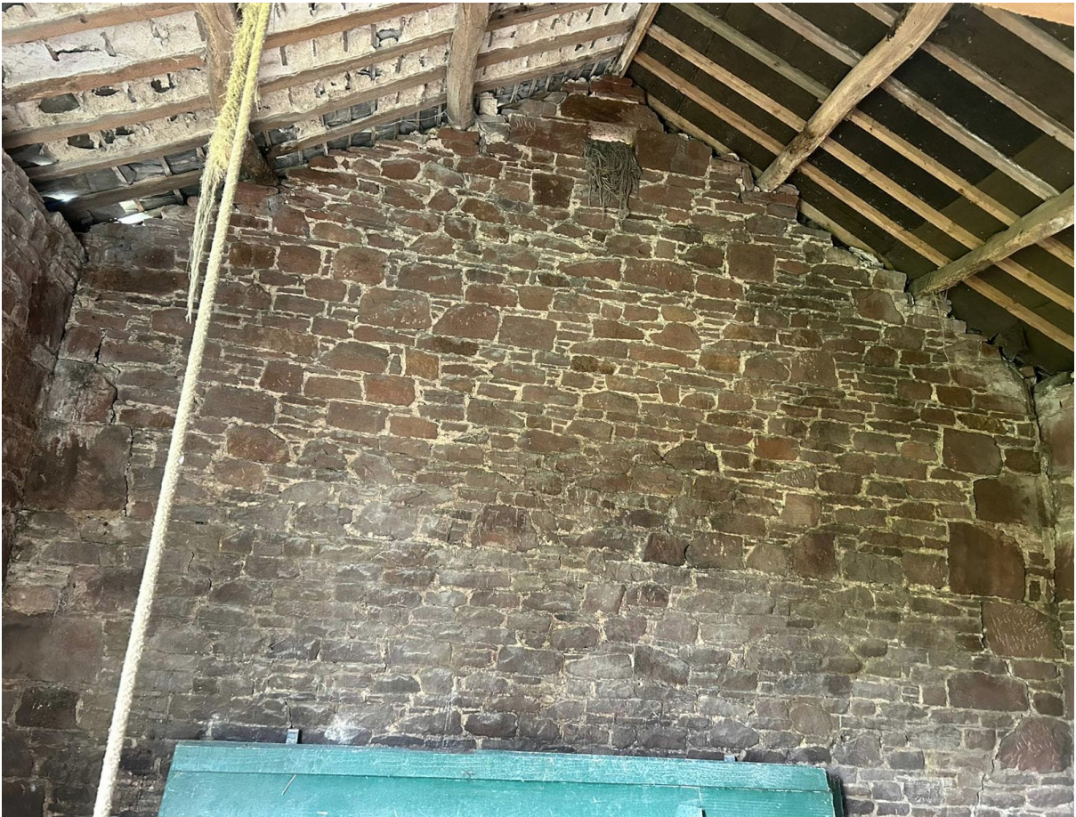
Fig 1 Photograph showing existing roof with repaired section.
