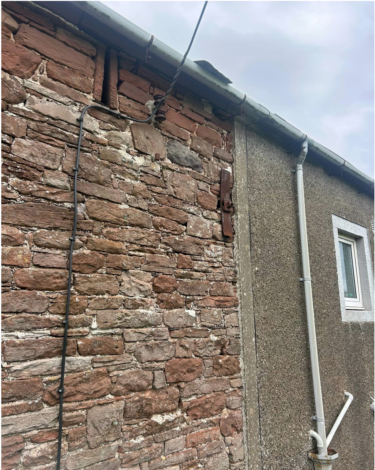
Fig 7 photograph showing external tie member plate on rear elevation
