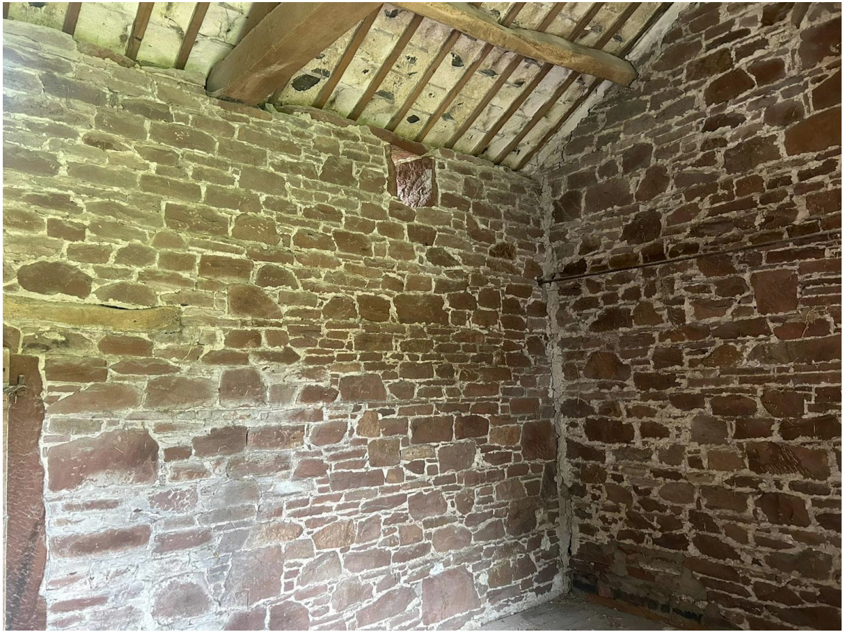
Fig 8 Photograph showing tie member within barn.
