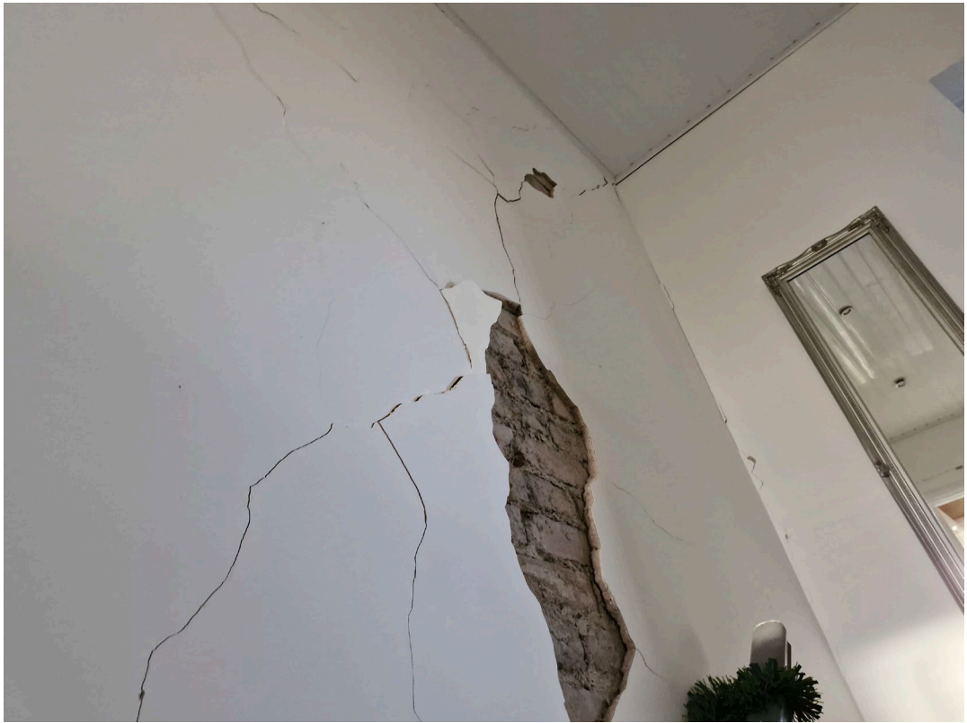
PHOTO 03 DAMAGE TO PARTY WALL No 27/28
