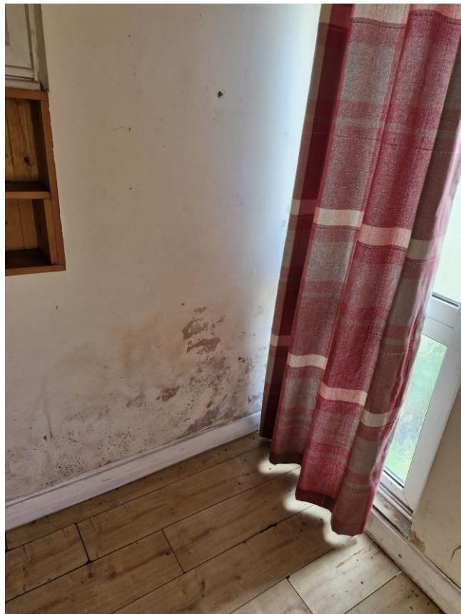
PHOTO 10 VIEW ON DAMP TO REAR EXTENSION
