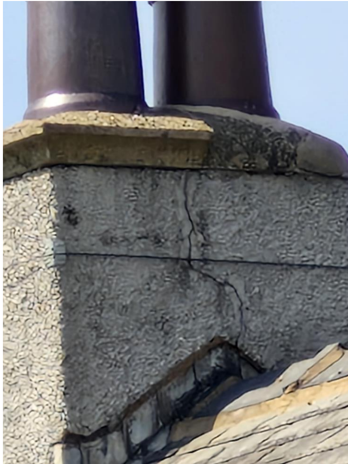
PHOTO 07 CRACK TO CHIMNEY STACK
