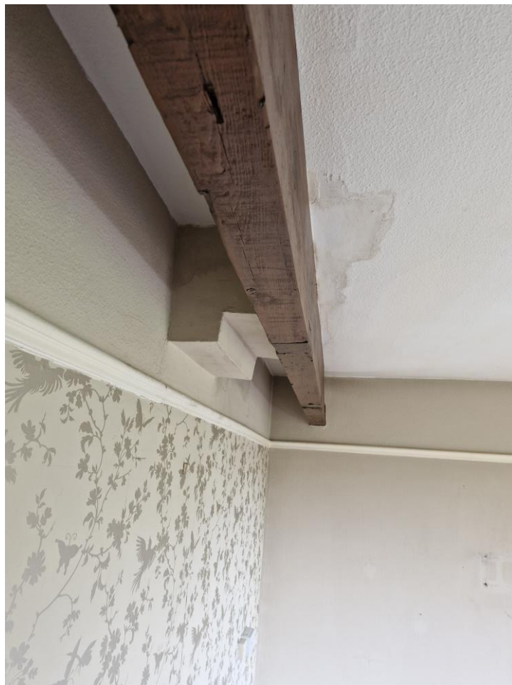
PHOTO 04 CHIMNEY BREAST SUPPORTS.
