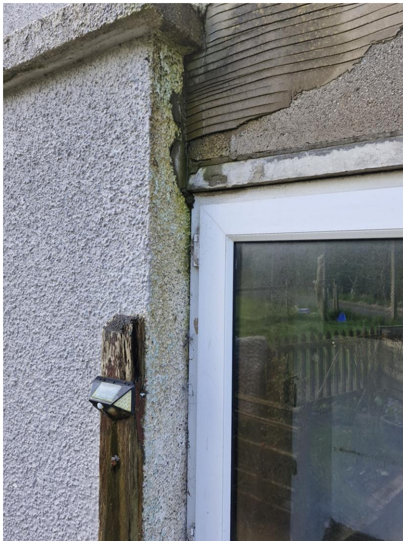
PHOTO 06 INADEQUATELY FLASHED IN REAR EXTENSION
