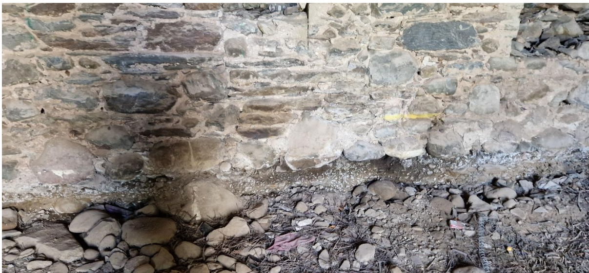
Photo 5 - Barn 3 - Excavations Below Foundation Stones
