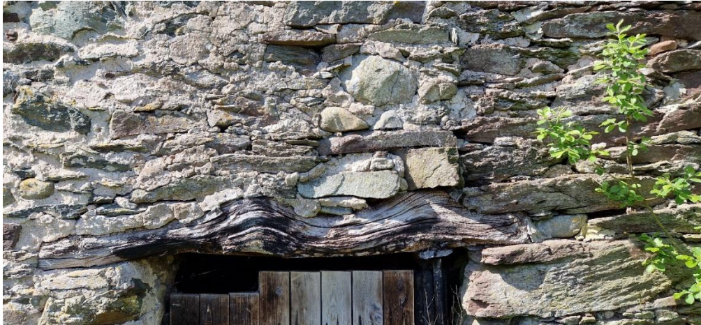
Photo 10 - East Elevation of Barn 2 - Movement Above Lintel
