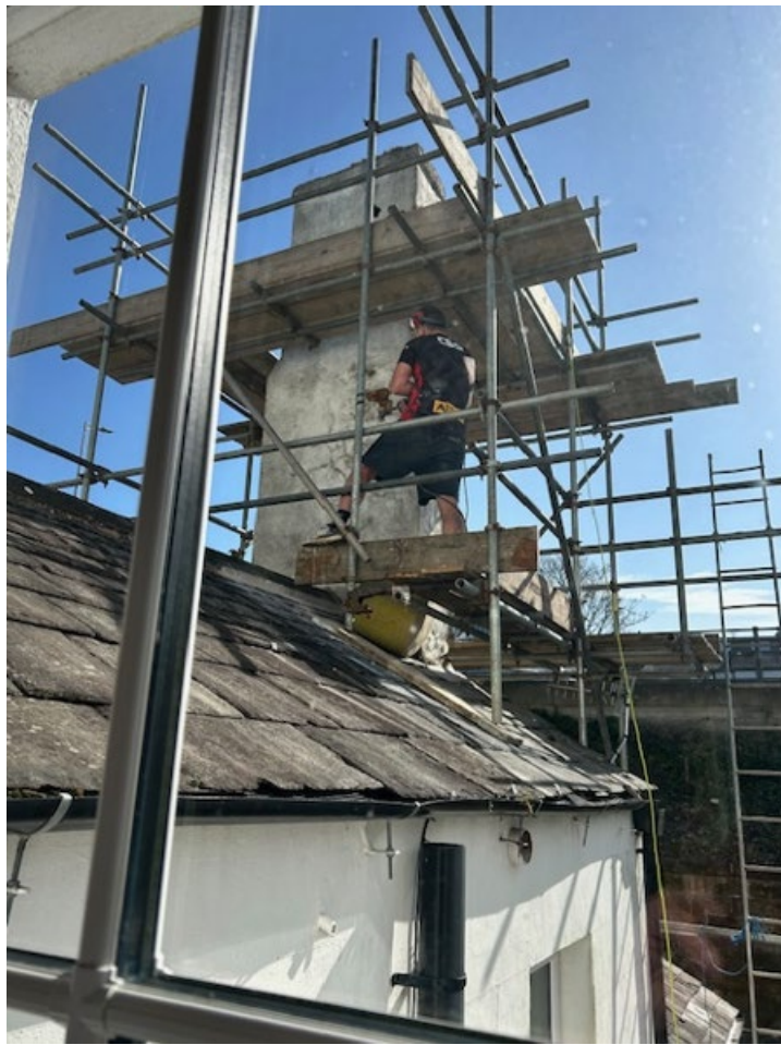
PHOTO 1 VIEW ON STACK
