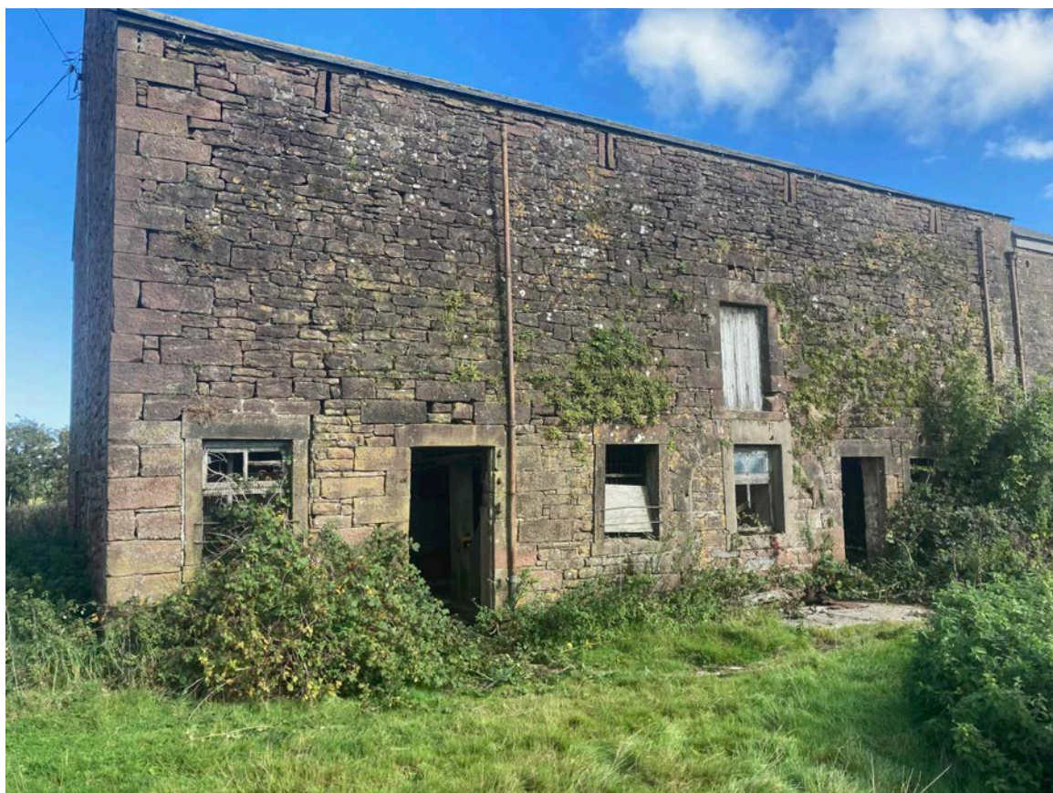
Photo 14 - South elevation of barn with outward bulging masonry
