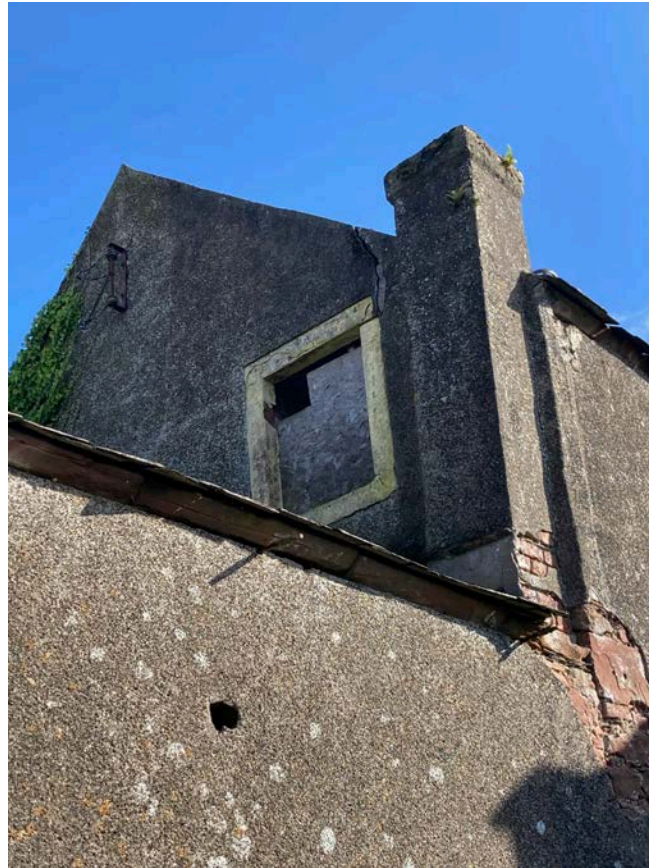
Photo 3 - North gable with vertical crack near window opening and failed cement render
