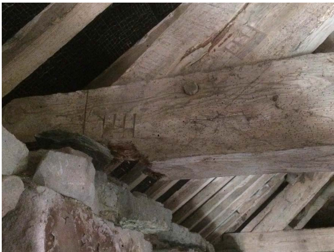
Photo 12 – Truss tie beam with rotten end
