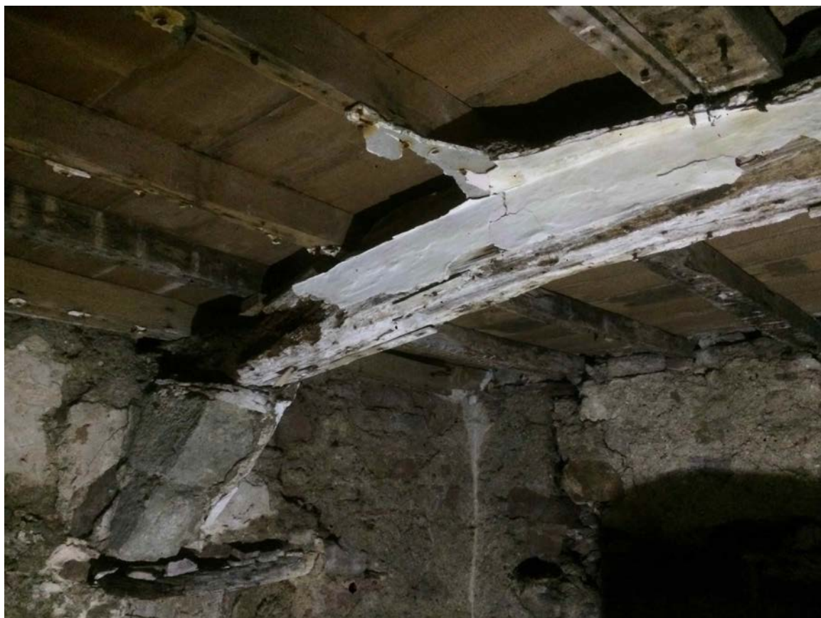
Photo 5 - Failed first floor timber beam over store
