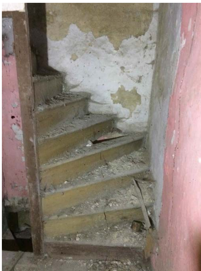
Photo 8 - Timber treads to second floor staircase in poor condition
