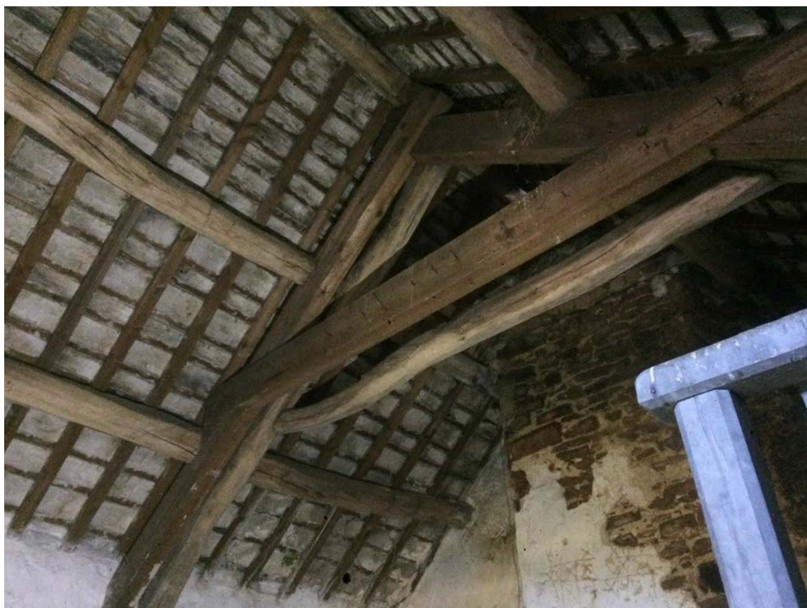
Photo 6 - Modern raised collar truss adjacent to original truss over service bedroom
