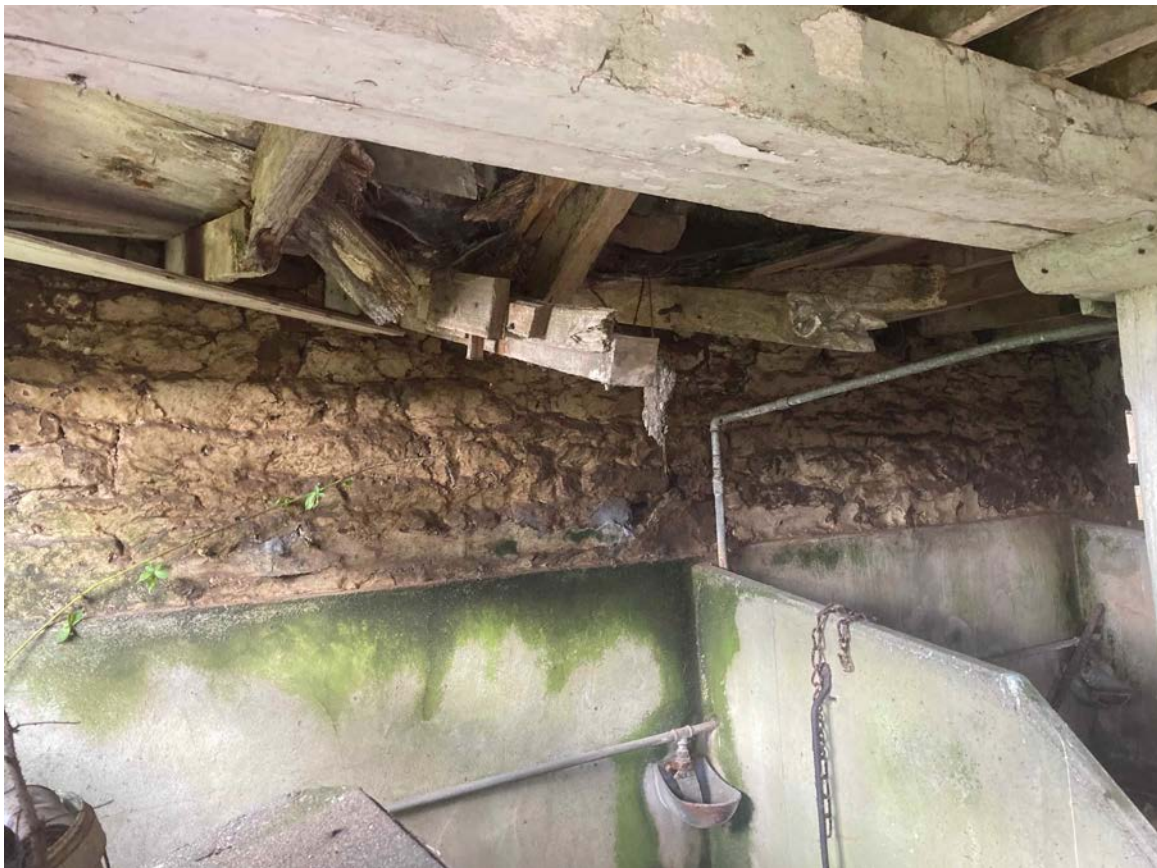
Photo 16 - Collapsed first floor joists in barn
