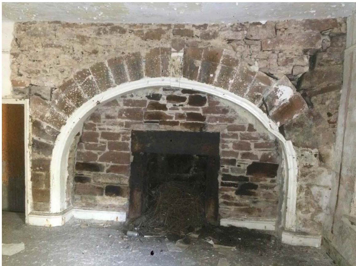
Photo 4 - Stone arch with shear failure to voussoir stone
