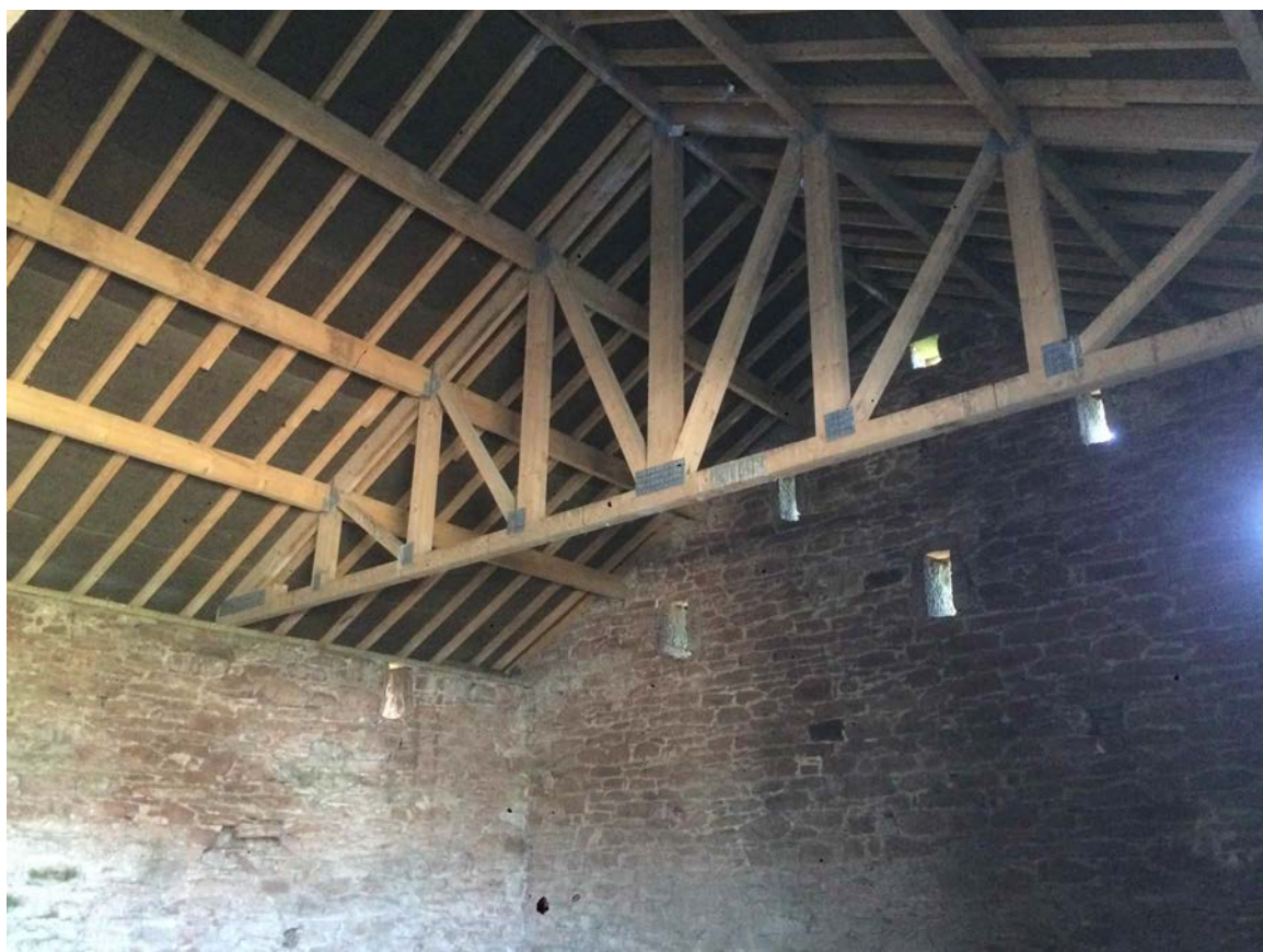
Photo 18 – Modern softwood roof trusses over barn
