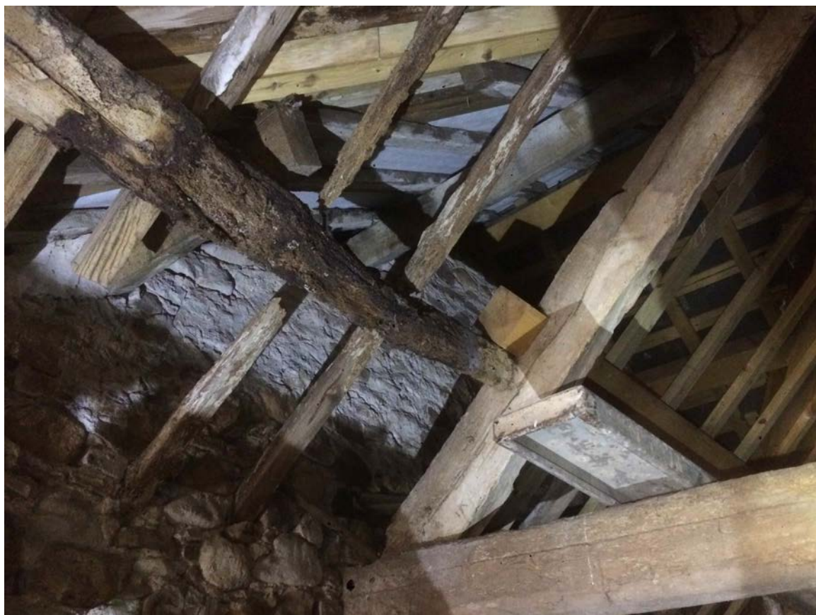
Photo 11 - Rotten purlin and common rafters
