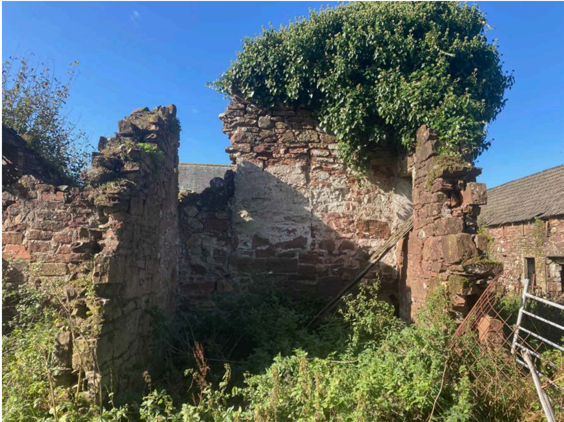
Photo 20 - Vegetation growth and exposed masonry wall heads to Outbuilding No. 2
