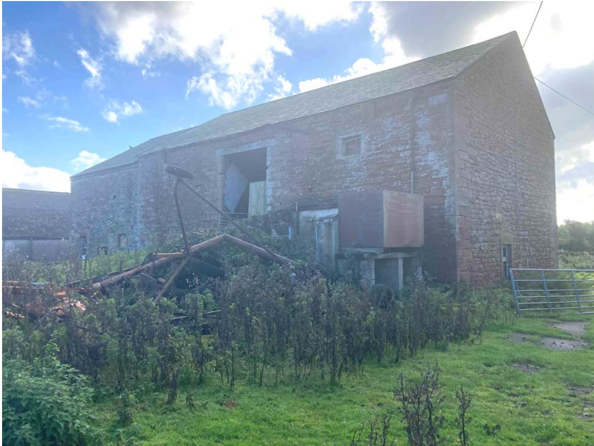
Photo 15 - North elevation of barn with rotten timber lintel over cart shed
