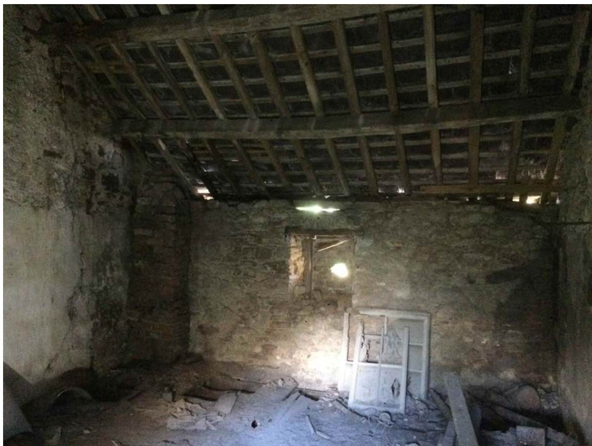
Photo 7 - Roof over link building with rotten purlin end
