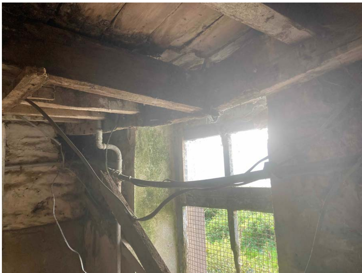
Photo 17 – Collapsed first floor joists and rotten wall plate
