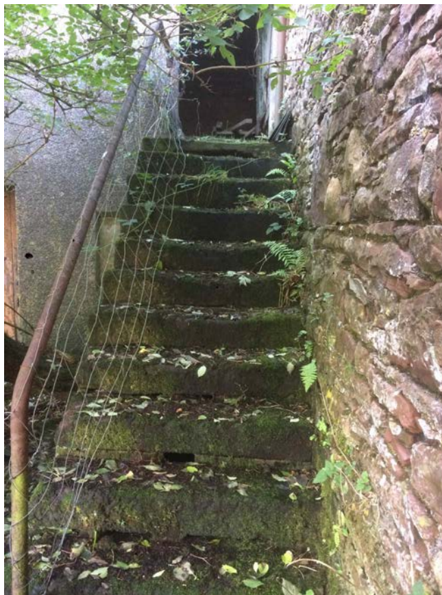
Photo 13 - External staircase with vegetation growth on treads and loose balustrade
