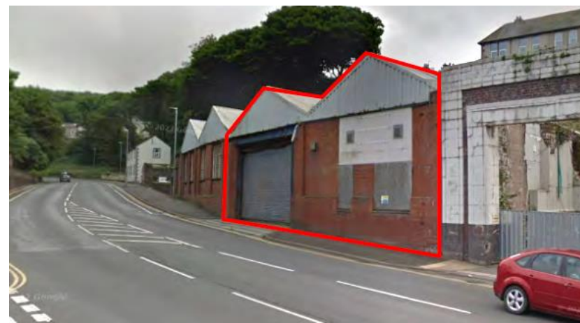
Figure 2 Street view of the former Warehouse from New Road
