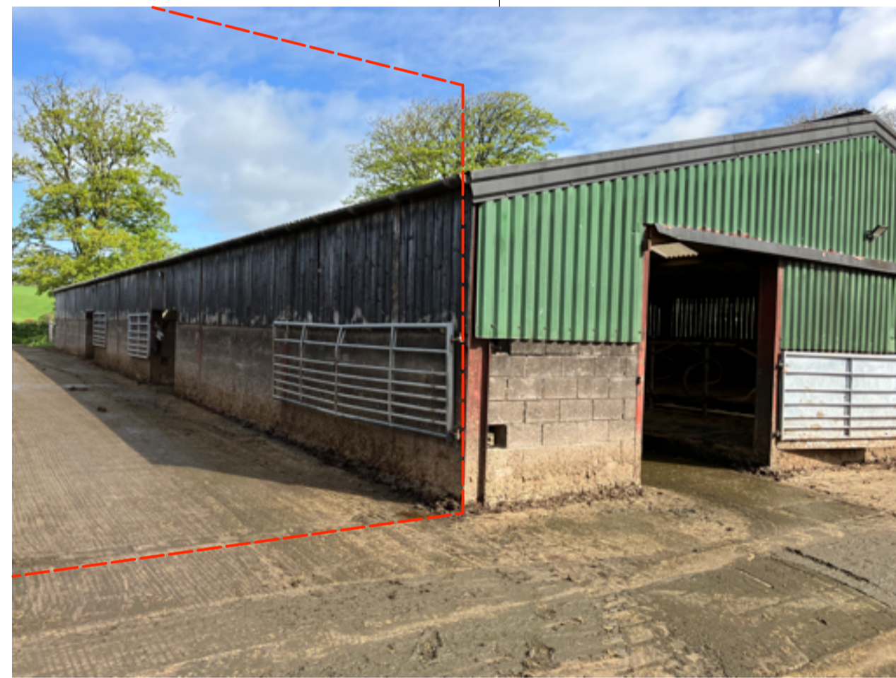
ROOF OVER PASSAGE
