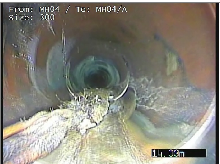
Roots mass 20% cross-sectional area loss, Start
