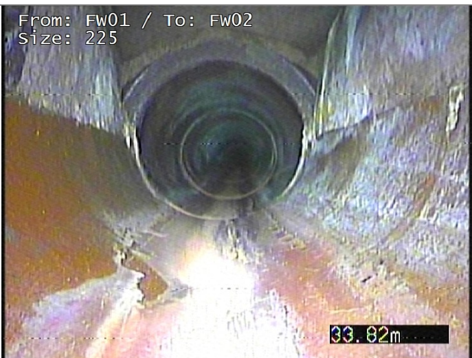
Finish node type, manhole, reference FW02
