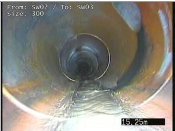
Junction at 2 o'clock, diameter 150mm
