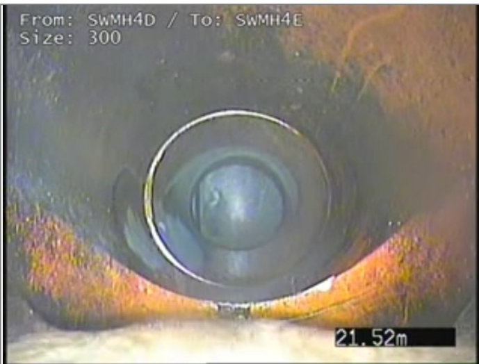
Junction at 6 o'clock, diameter 300mm - Remark: BACK DROP CONNECTION TO SWMH4E
