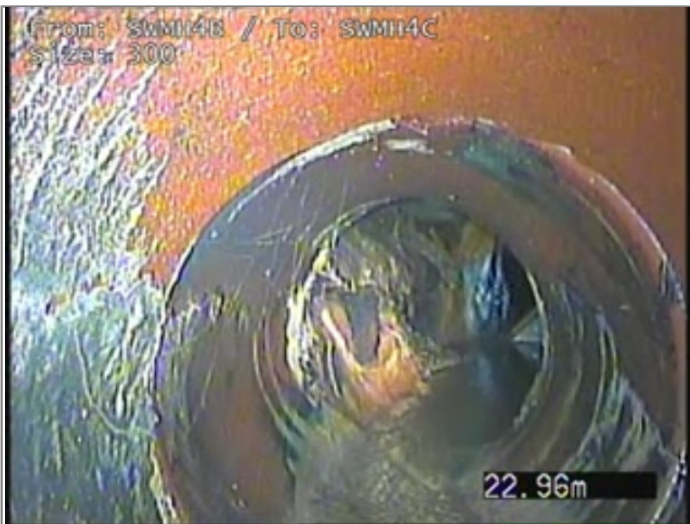
MANHOLE VISIBLE IN THE DISTANCE.
