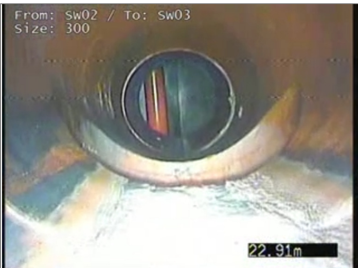
Junction at 6 o'clock, diameter 300mm - Remark: BACK DROP CONNECTION TO MANHOLE
