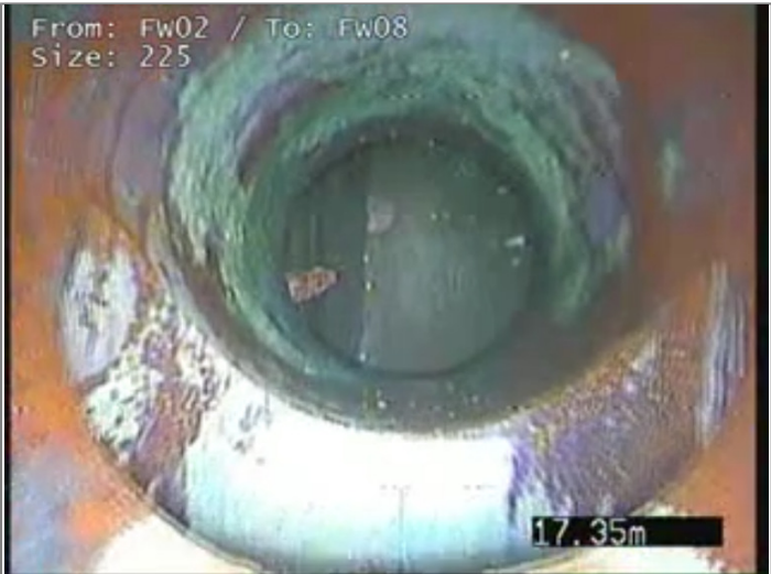
Junction at 6 o'clock, diameter 225mm - Remark: BACK DROP CONNECTION TO MANHOLE
