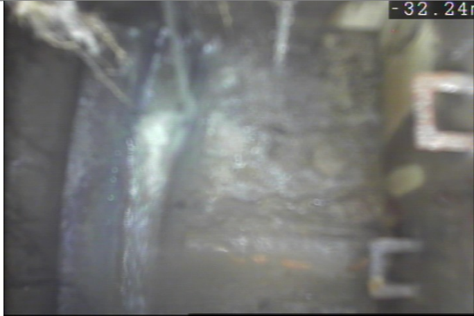
Manhole / Access Point: FWMH13A Internal
