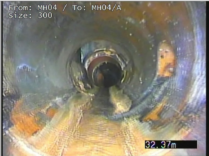
Junction at 3 o'clock, diameter 100mm
