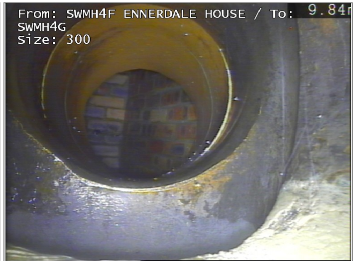
Finish node type, manhole, reference SWMH4G UNDER SANDBAGS
