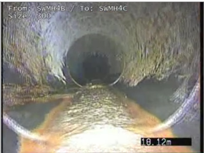
Roots tap at joint - Remark: 8 OCLOCK
