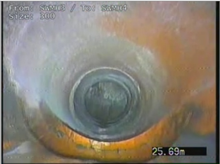
Junction at 6 o'clock, diameter 300mm - Remark: BACK DROP CONNECTION TO SWMH4
