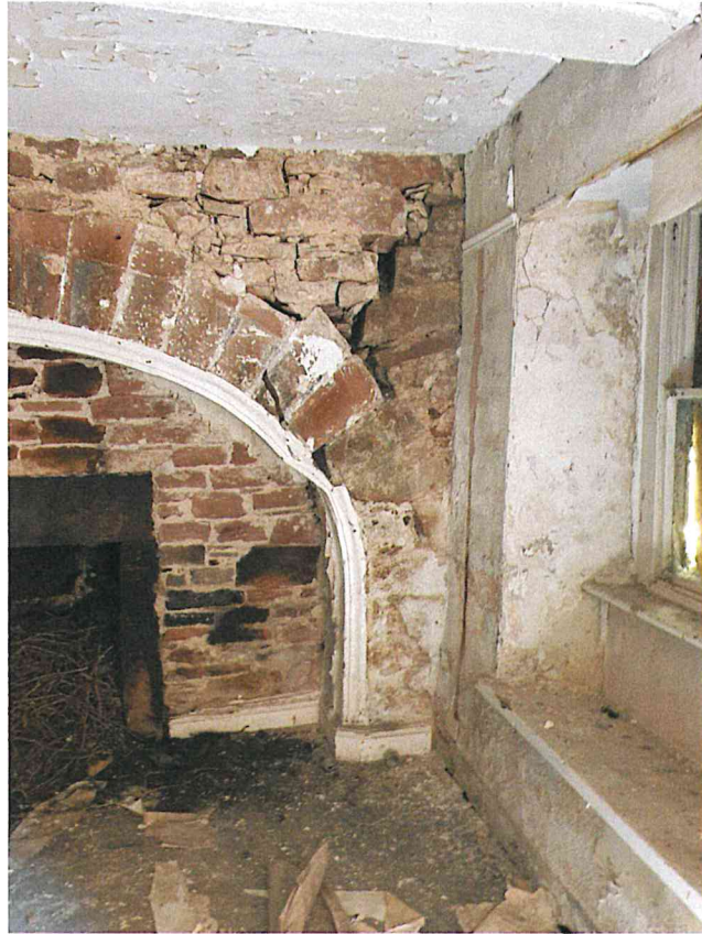
PHOTO 01 VIEW ON FRONT WALL BOW & MOVEMENT TO INNER WALL
