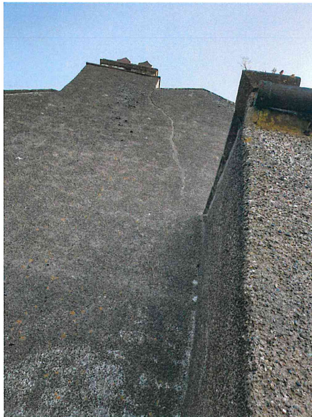
PHOTO 4 VIEW ON CRACK TO REAR ELEVATION MAIN HOUSE.
