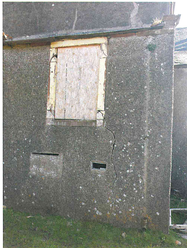
PHOTO 02 VIEW ON CRACKING TO REAR ELEVATION EXTENSION
