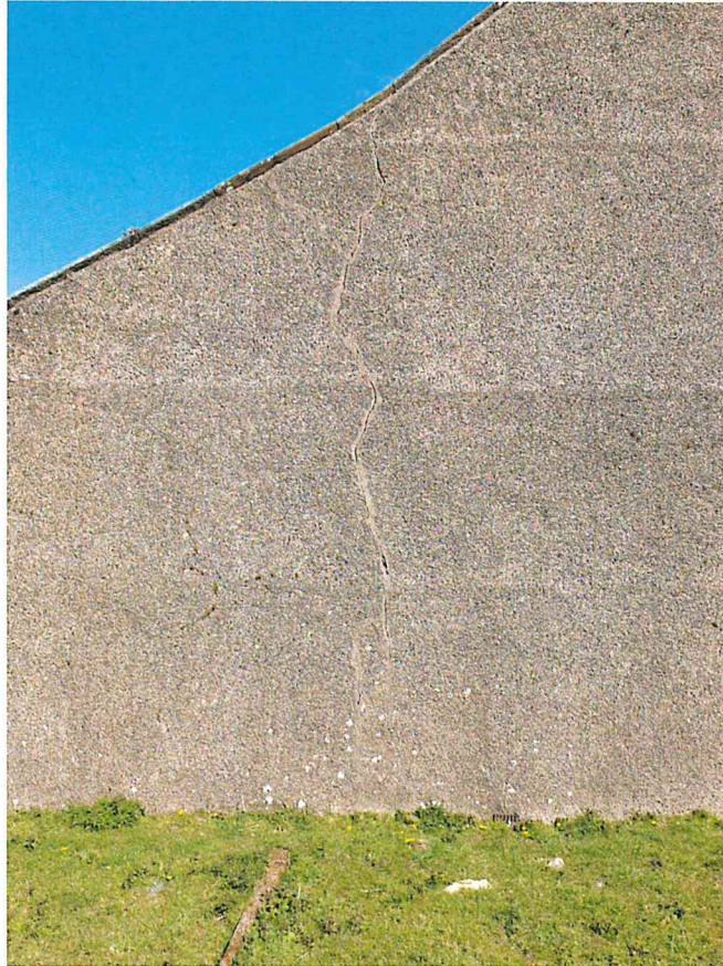
PHOTO 03 VIEW ON CRACKING TO LEFT HAND ELEVATION
