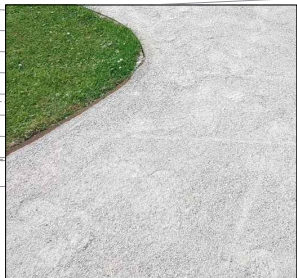
Main path through site built with grey Hoggin Self Binding Gravel 10mm to dust.
