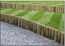
250mm diameter wooden post retaining wall.
