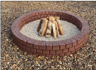
120 cm brick fire pit made from fire bricks. Or similar approved.
