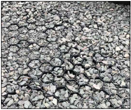
Gravel surface for parking area. Permeable gravel grid.
