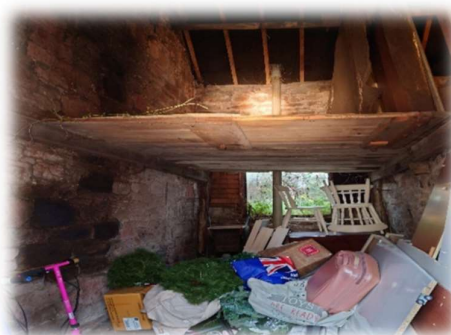
Plate 10: Ground floor used for storage.
