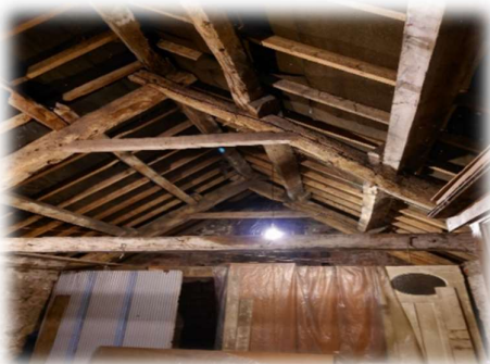
Plate 9: Internal roof void.
