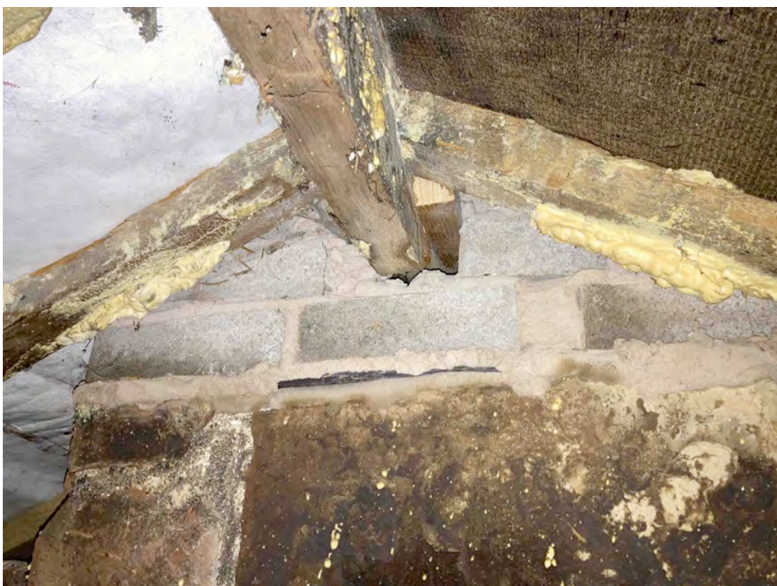
Photo 02 – Ridge beam inadequately supported at end bearing.
