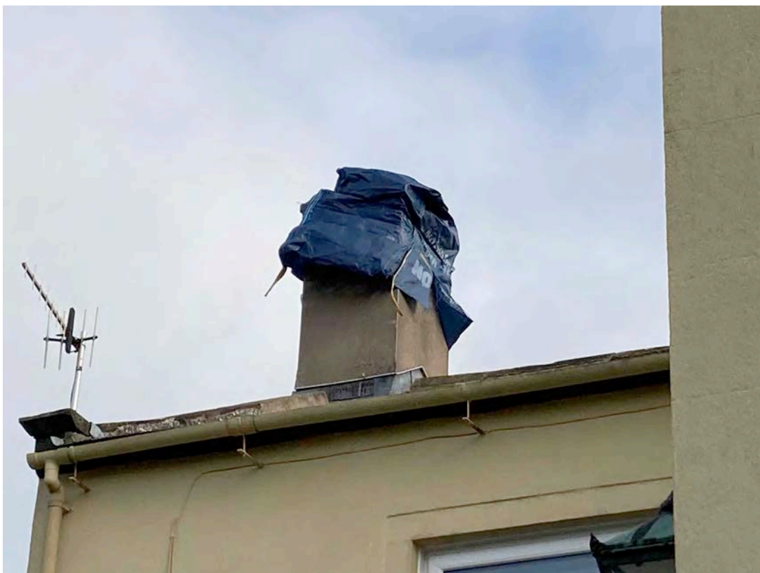
Photo 03 – Rebuilt chimney stack in blockwork with cement render (Nov 2021)
