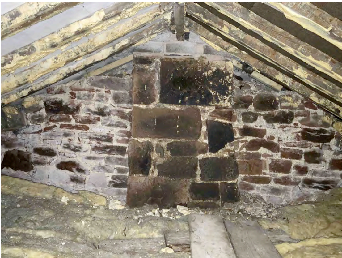
Photo 01 – Stone chimney breast with 2 no. courses of blockwork within attic space.
