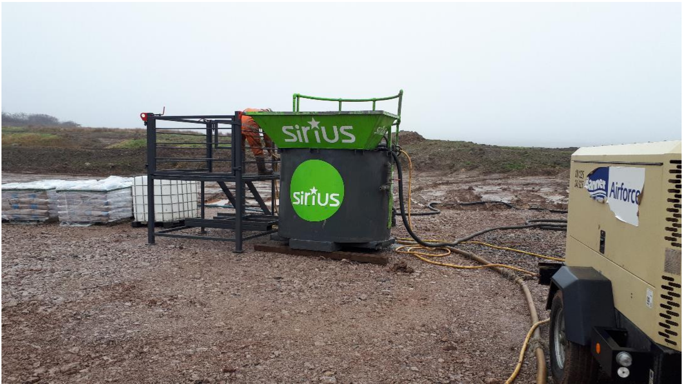
Photograph 3: Grout mixer, platform, compressor and OPC stockpile.
