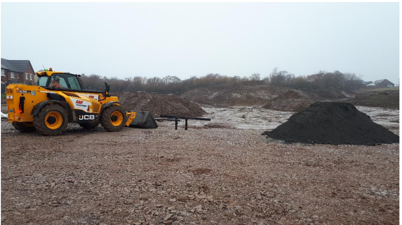
Photograph 4: Telescopic loader and delivery 1 of PFA.
