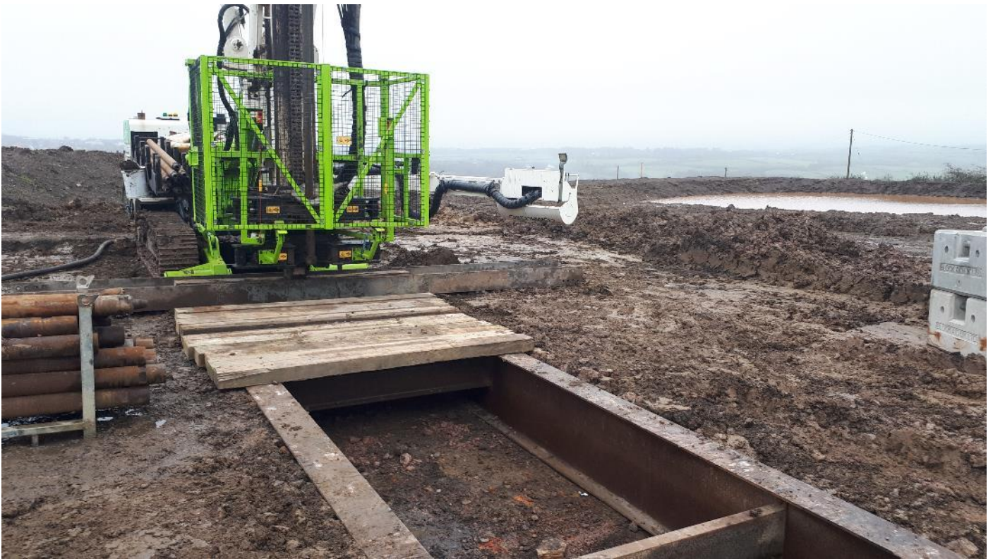
Photograph 1: Rig setup over shaft using shaft safety platform.
