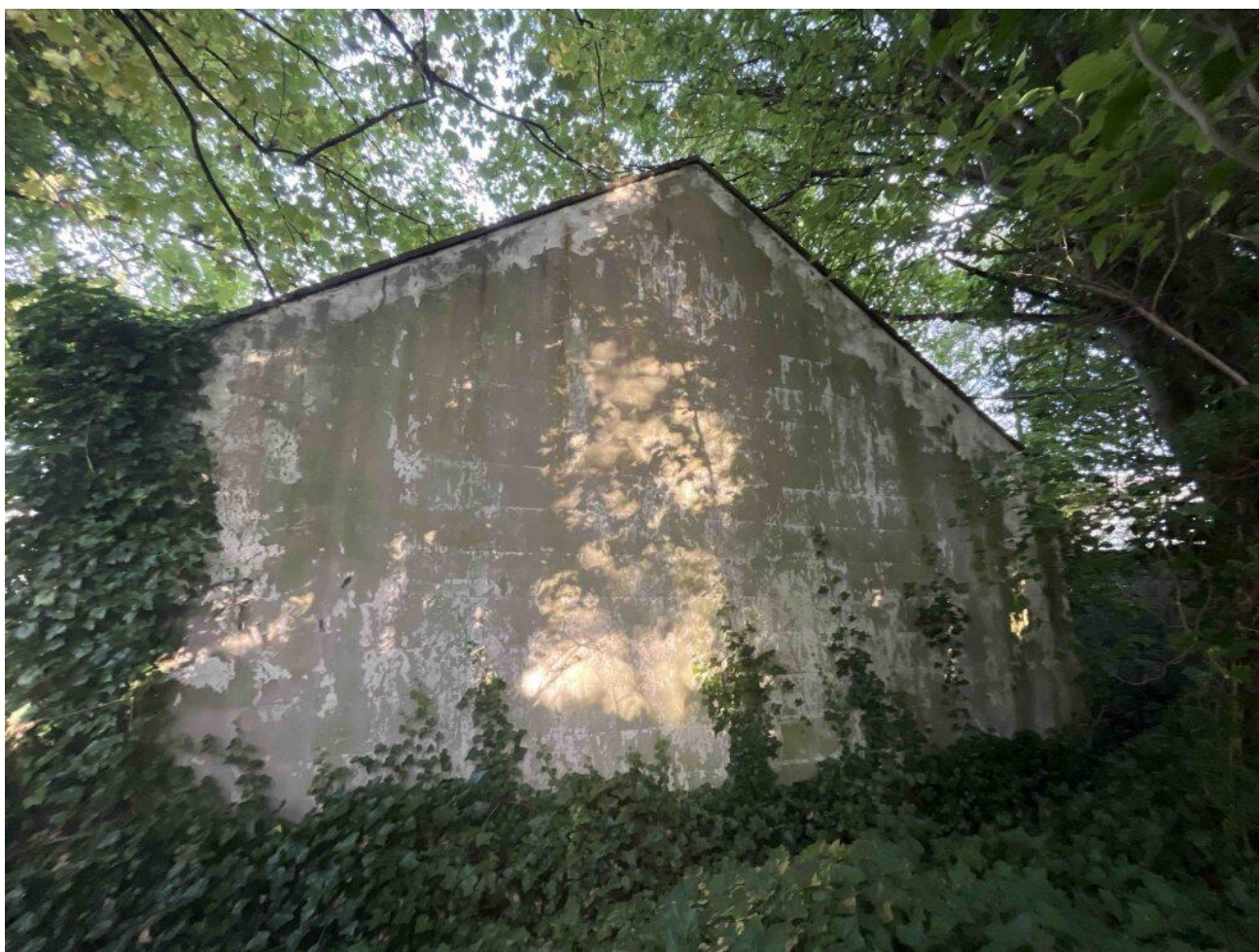
Image 7 – Rear aspect of building
