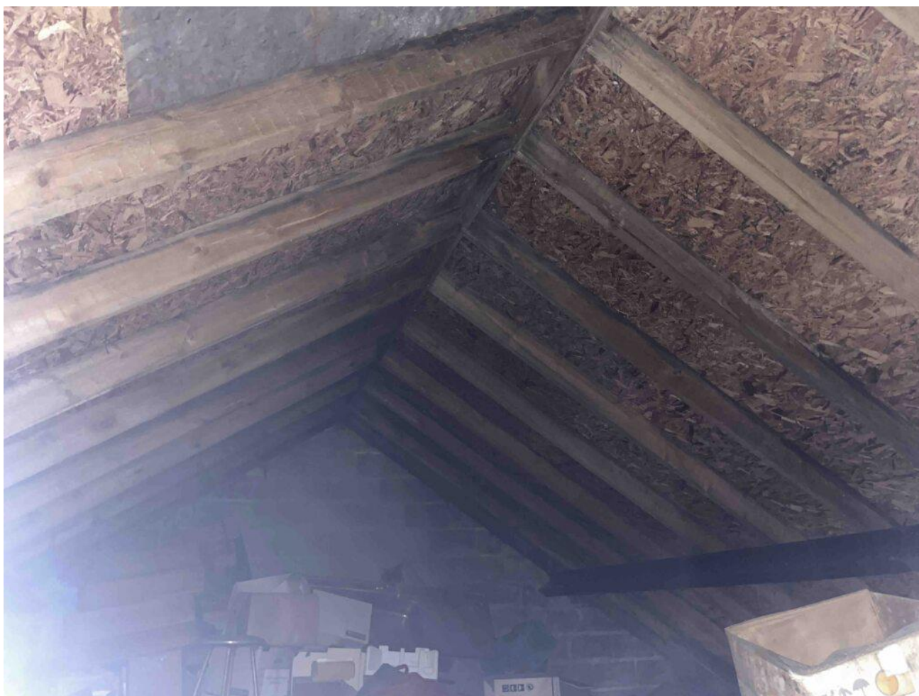
Image 8 – Internal roof space
