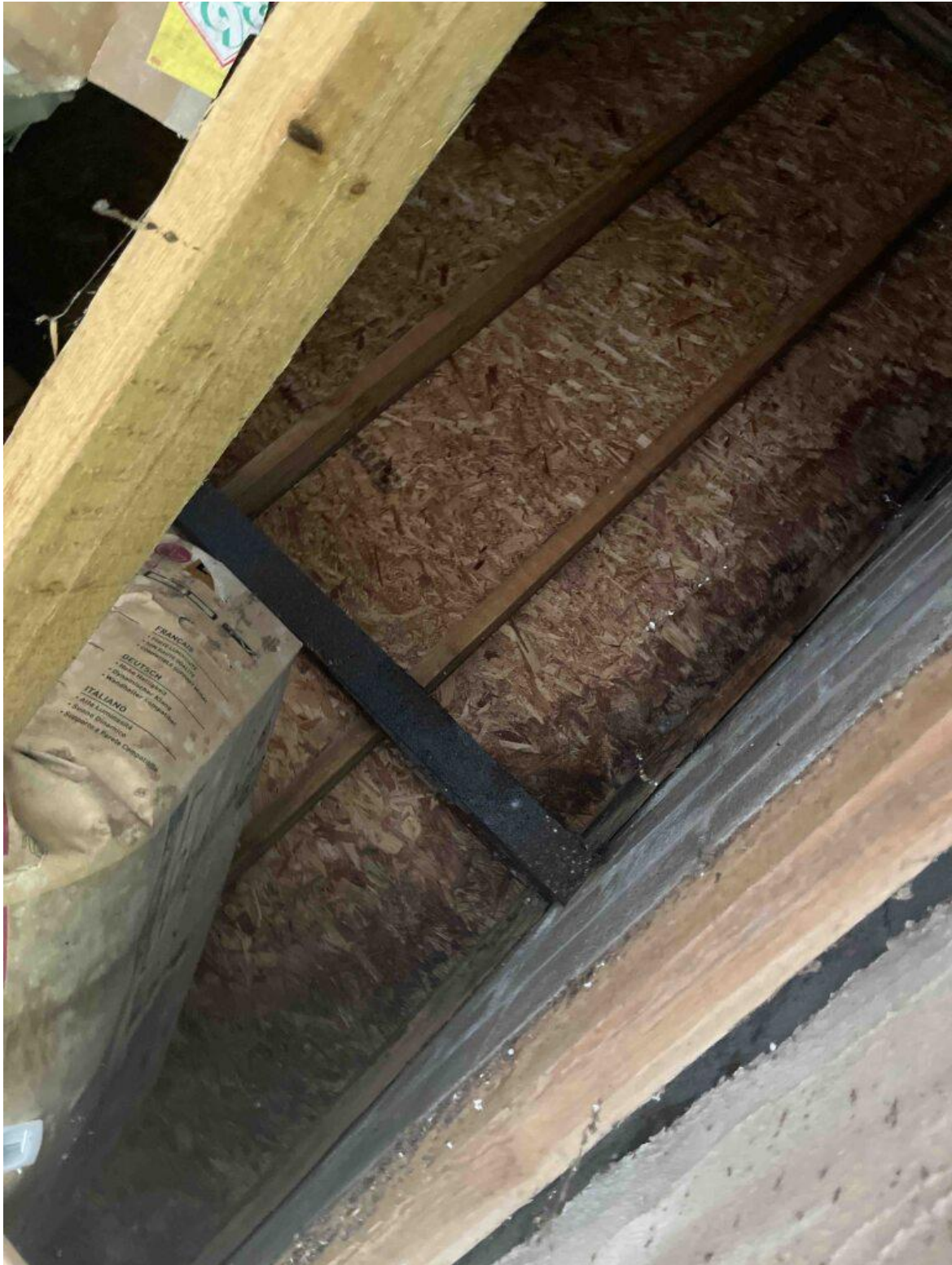
Image 3 – Internal aspect of roof
