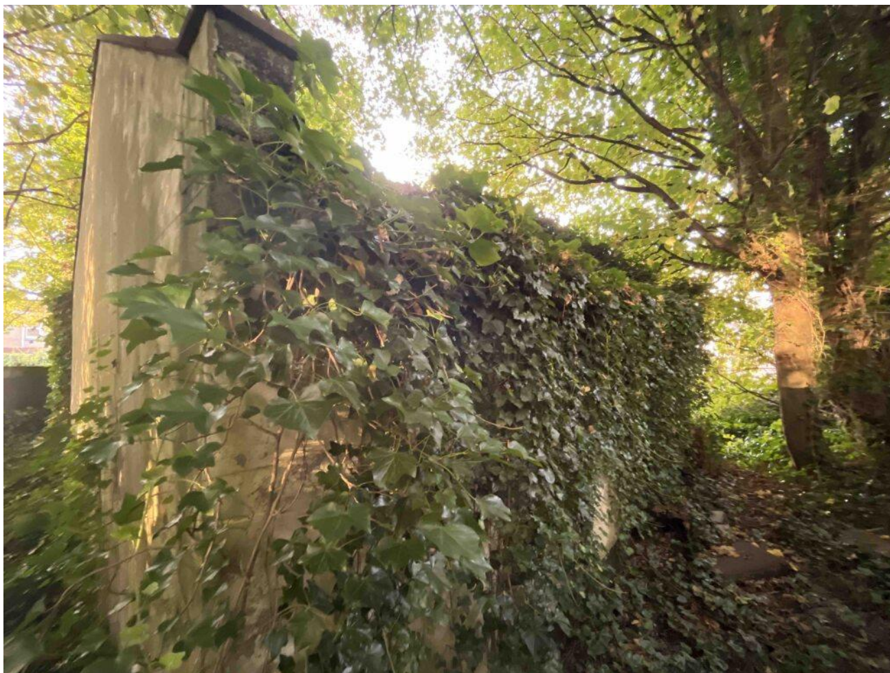
Image 6 – Side view of building, thick covering of ivy – potential roosting feature
