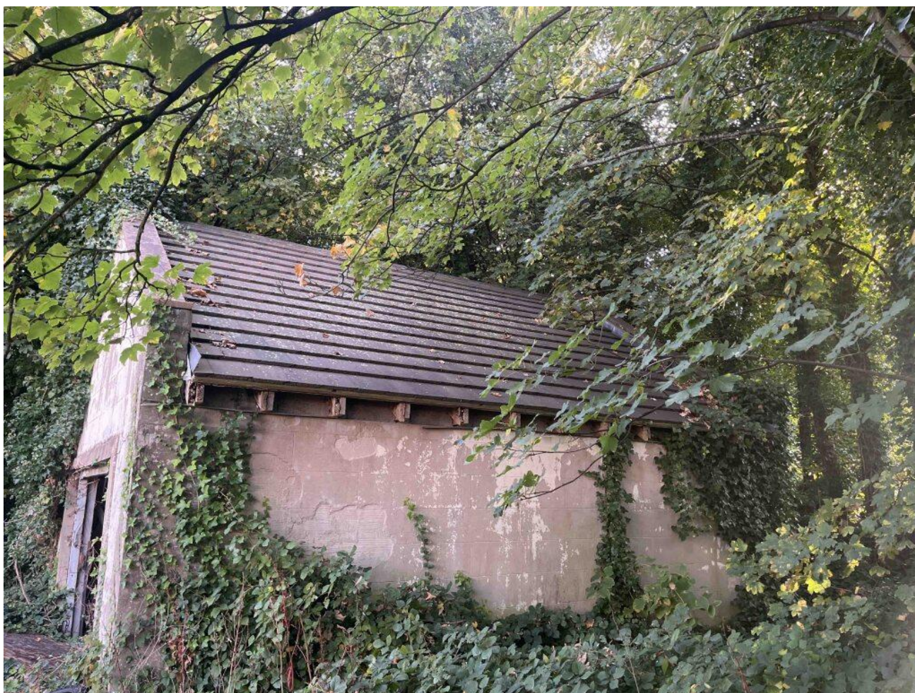
Image 5 – Side view of building
