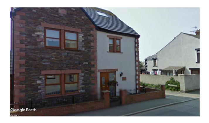
Proposed external materials are made up as follows (example above of a local property on Main Street, Haverigg, <u>for which all quoins and lintels are to be in Lakeland slate and not sandstone</u>):
