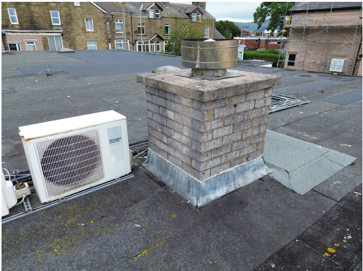
4 – Lead flashing is fitted tightly around chimneys and flues with no suitable gaps.
