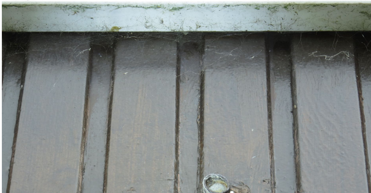
5 – Fascia boards are fitted tightly against cladding with no suitable gaps.
