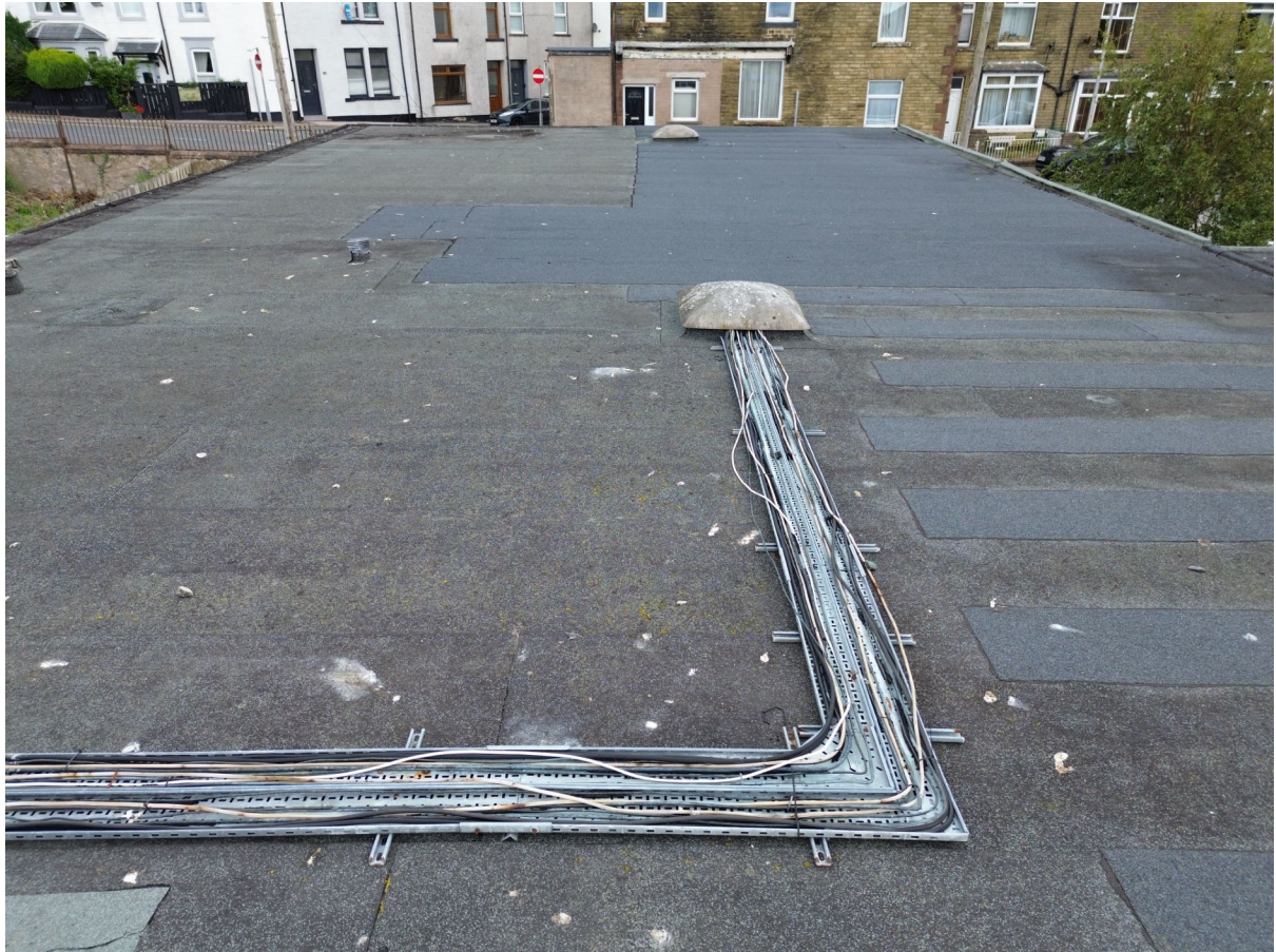
3 – The roof is in generally good condition with no obvious gaps between materials.
