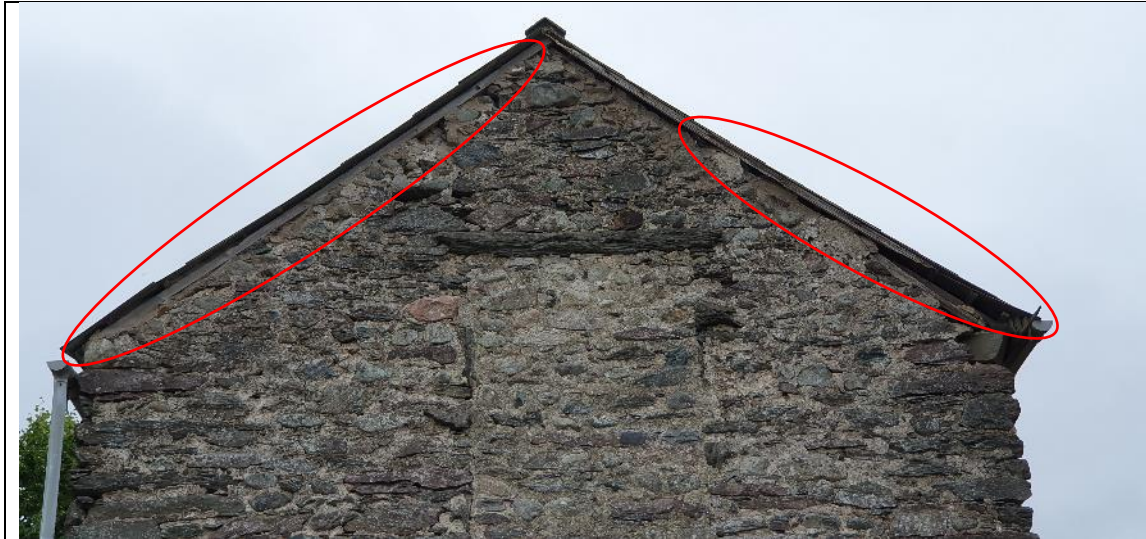
B1a southern gable end with gaps between wall tops and roof verge
