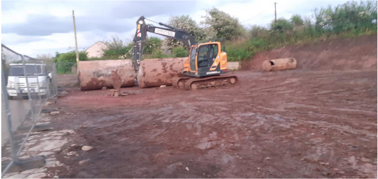
IMAGE 3 – TAKEN LOOKING EAST AFTER DEMOLITION & SITE CLEARANCE.
