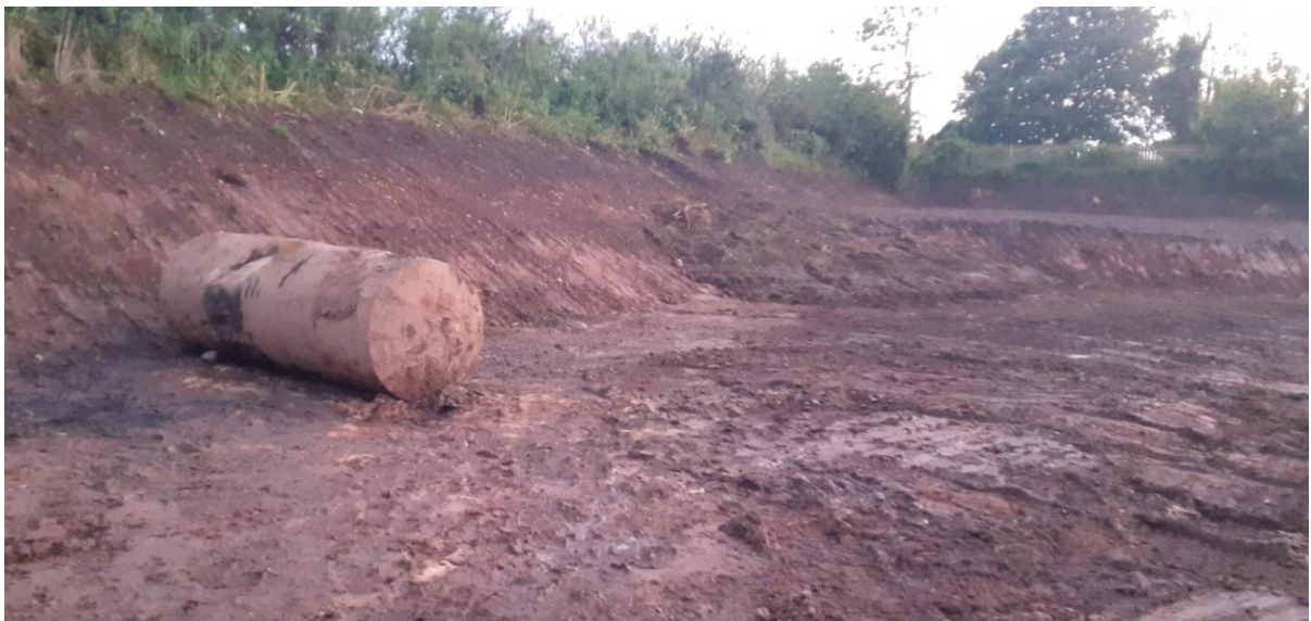
IMAGE 4 – TAKEN LOOKING SOUTHWEST AFTER DEMOLITION & SITE CLEARANCE.
