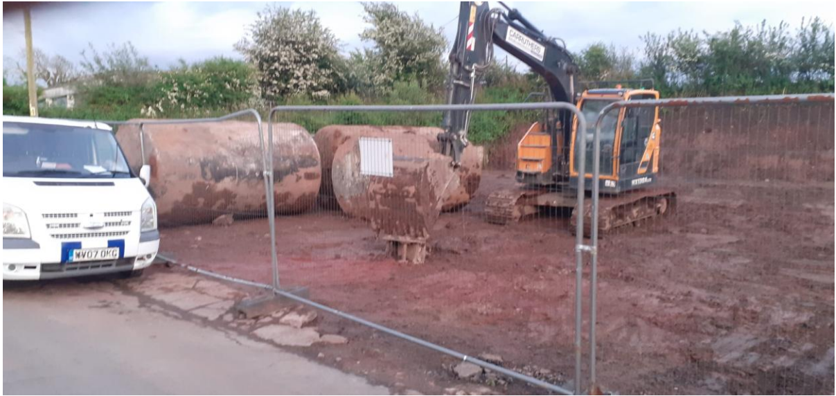
IMAGE 1 – TAKEN FROM PUBLIC HIGHWAY LOOKING SOUTHEAST AFTER DEMOLITION & SITE CLEARANCE.
