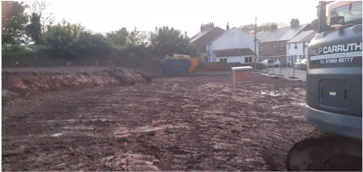
IMAGE 5 – TAKEN LOOKING WEST AFTER DEMOLITION & SITE CLEARANCE.
