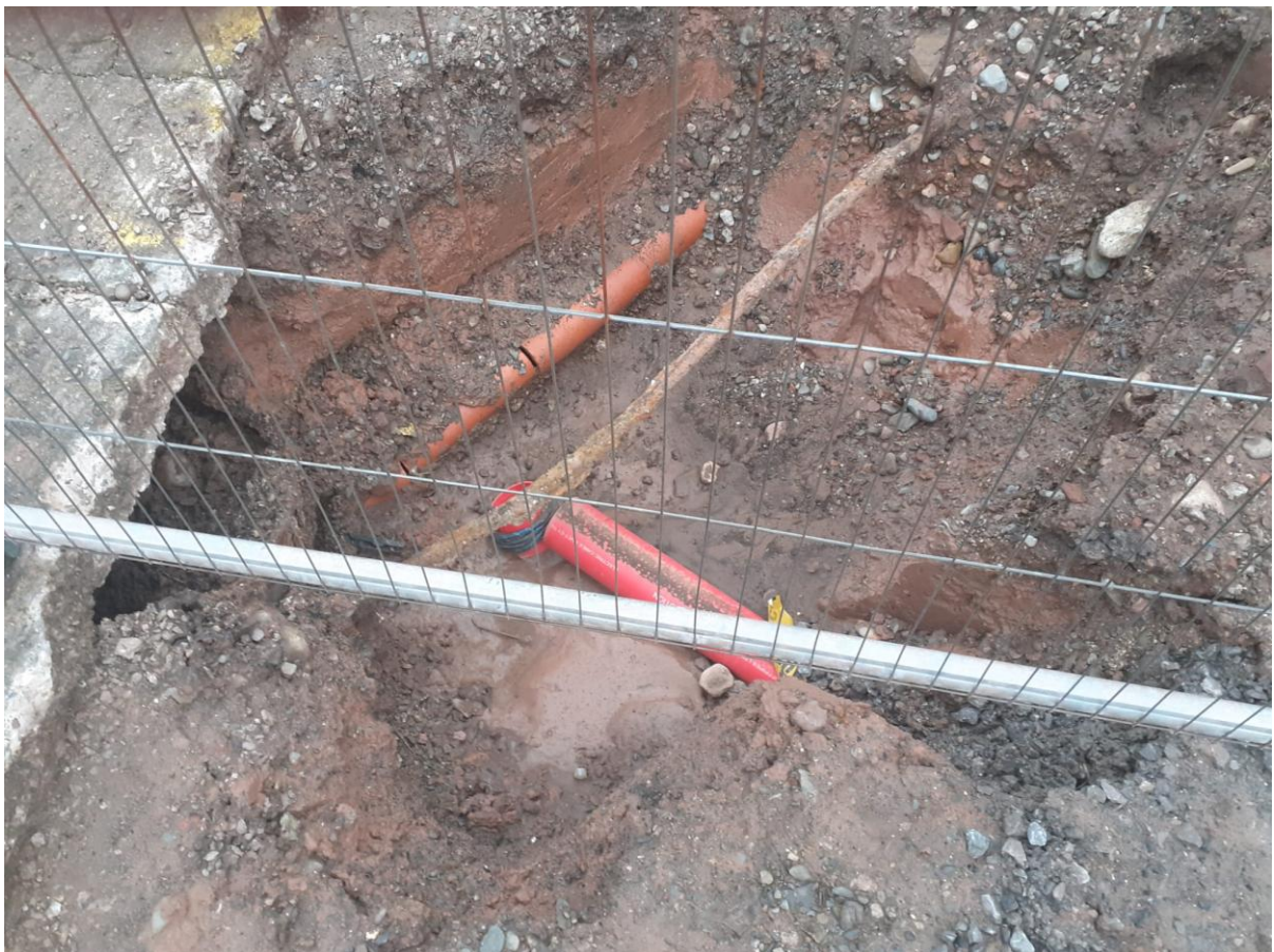
IMAGE 2 – EXCAVATION SHOWING EXISTING SERVICES TAKEN DURING DEMOLITION & SITE CLEARANCE.
