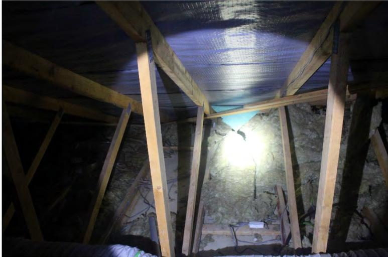
The roof voids in the clubhouse have timbers in good condition, and are relatively cluttered with struts. The roof lining is intact and the eaves lines are sealed. No signs of bats were found.
