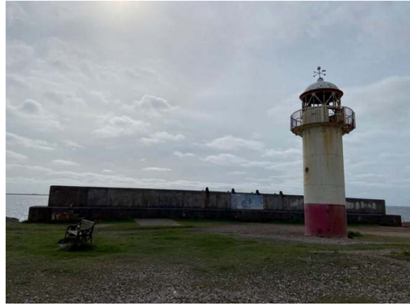
Photograph 2: Lighthouse and wall at the middle of the seawall
