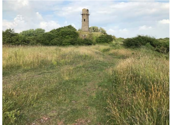
Photograph 2: General character of grassland habitats and the stone lighthouse
