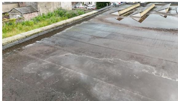
Photo 11: B1, sealed flat roof holding water
