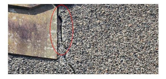
Figure 4 – crack in rendering on eastern elevation of B1.
