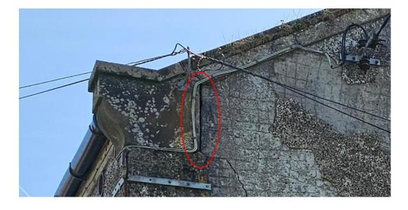
Figure 6 – crack in rendering on western elevations of B1.
