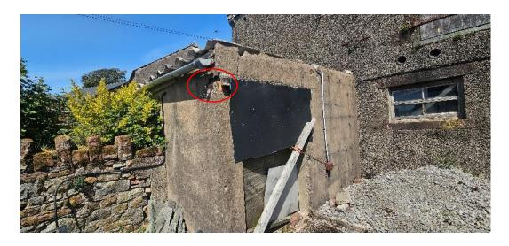
Figure 8 – crack in rendering on mono-pitch section on southern elevation of B1.
