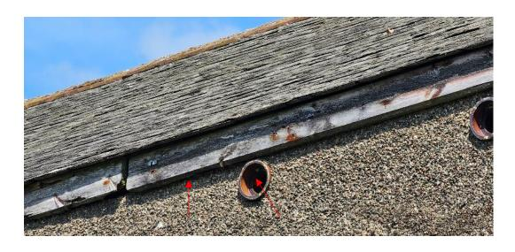
Figure 2 – gaps under soffits and pipes leading into interior on southern elevation of B1.
