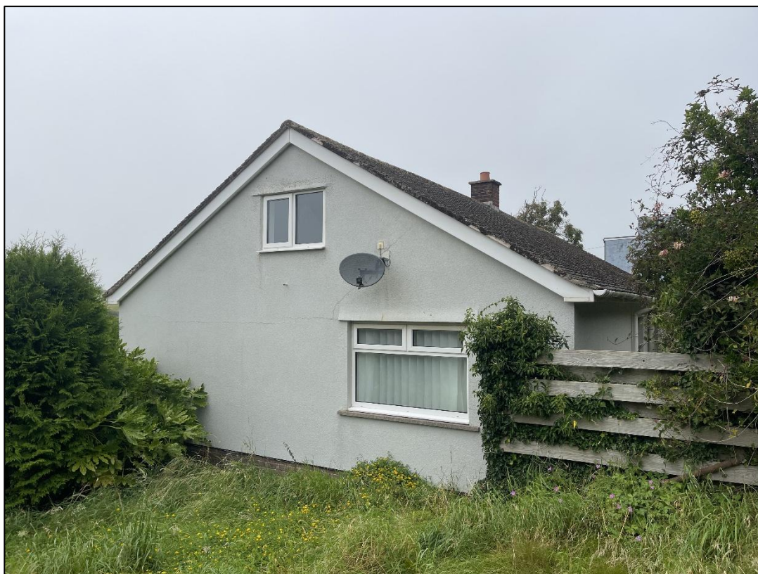
Plate 4 – Southern aspect of B1
