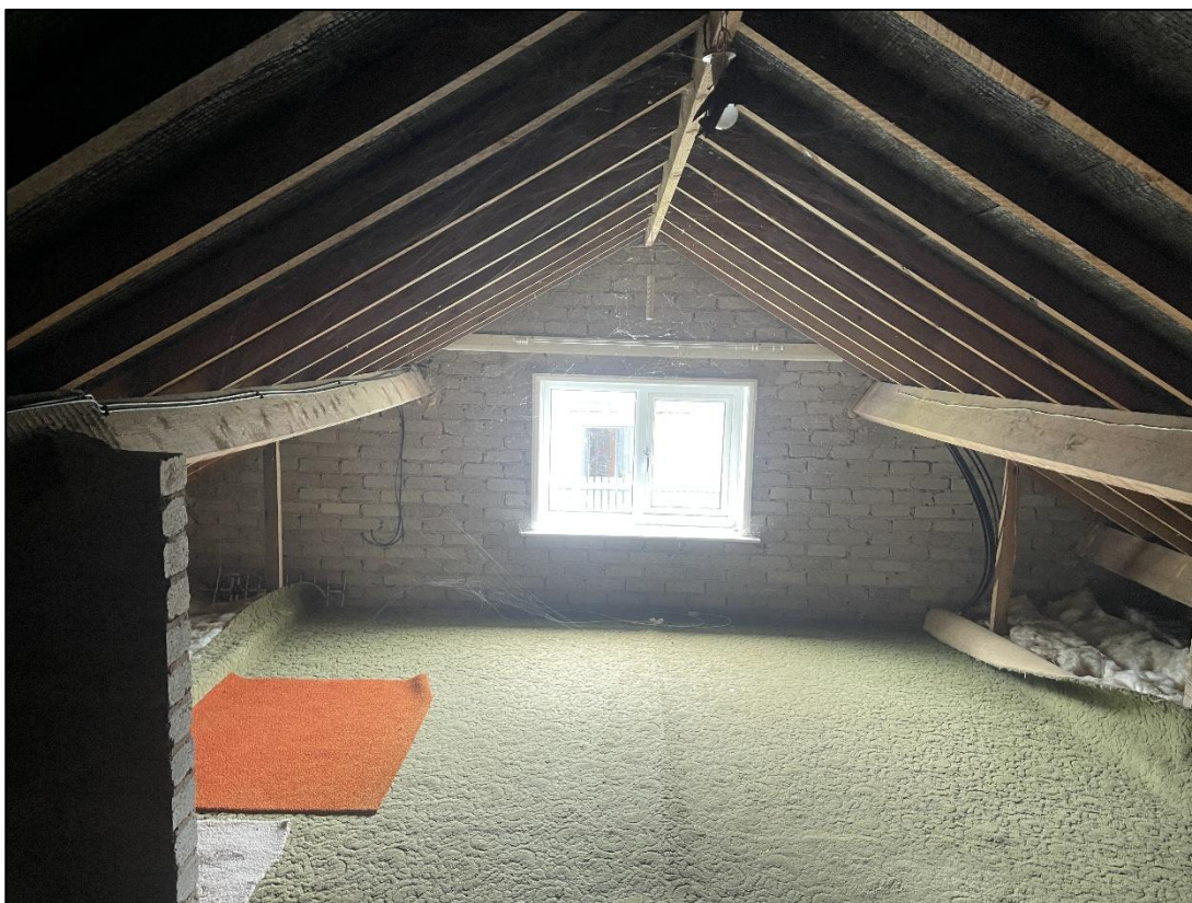
Plate 7 – Window at southern end of loft space
