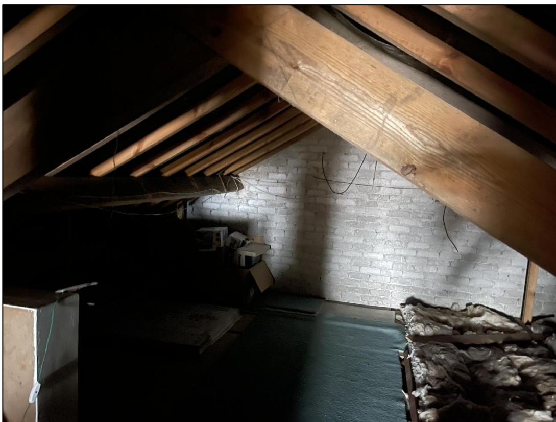
Plate 8 – Northern end of loft space, showing dark recesses
