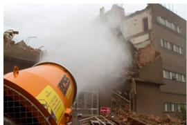
reduced down to first floor slab level. This process will continue systematically along the building leaving in the front as long as possible to create a screen to control the dust omissions. The front wall will then be brought inwards onto the building slab .A second excavator will work alongside the machine segregating waste streams for recycling. The process will be repeated for each bay along the length of the building.
