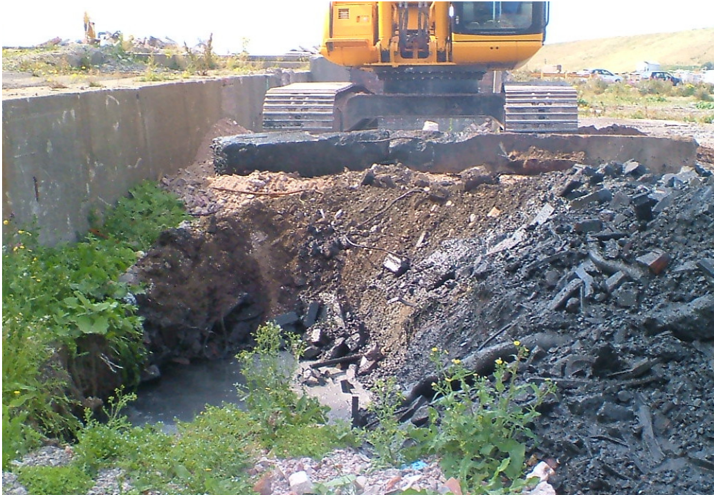
TP675B – black, oily perched ground water fills trial pit at 1.0m
