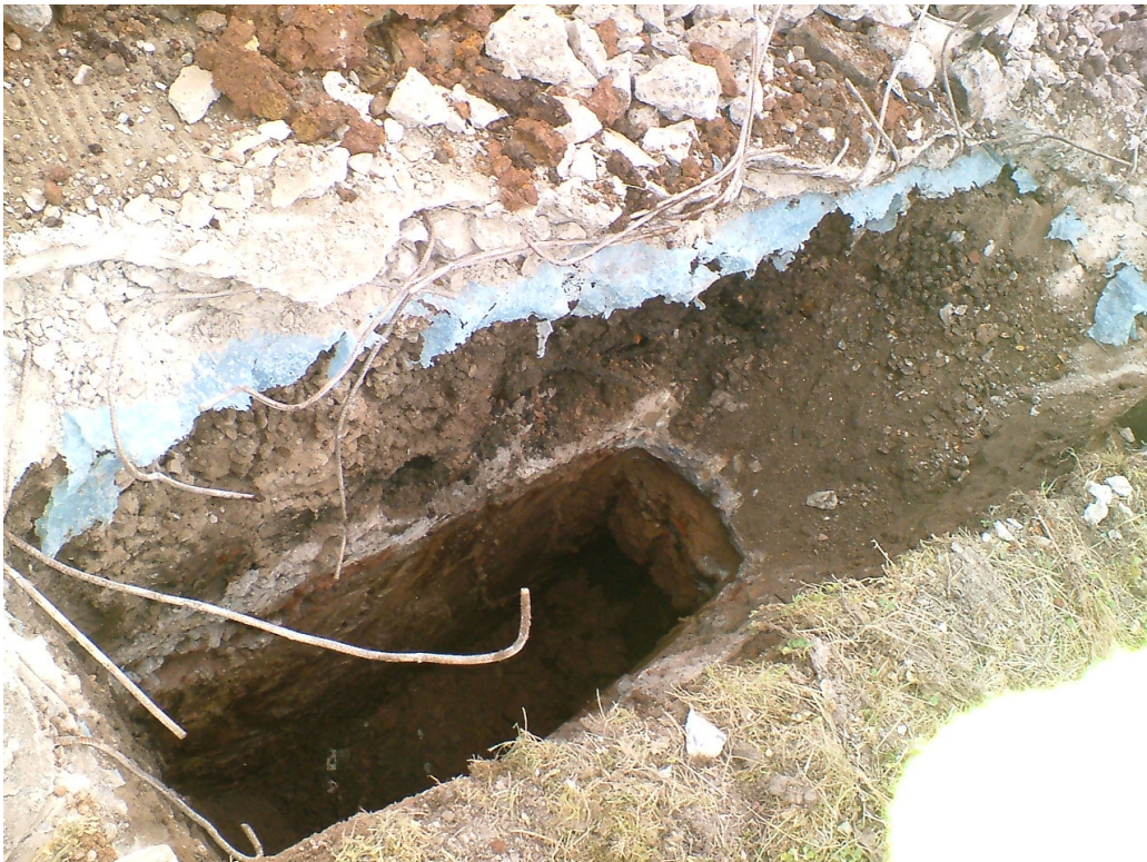
Photo 6 - TP616A –located in Plant Area, deep concrete foundations present at 1.0m bgl
