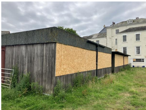
Above: the boarded up rear wing to be renovated and improved
