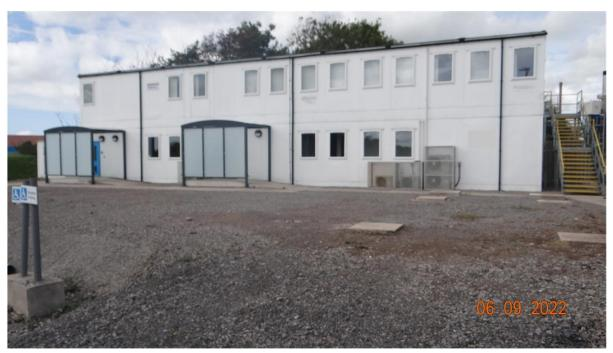
The proposed new 2-storey modular building will be of a similar modular construction type and colour (light grey) (see drawing HD/12889/01). New concrete footings (9 in total) will be required to support the building and they will be constructed on the existing compacted hardcore.
