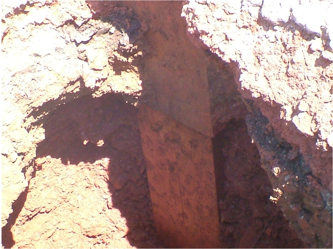
BH712C (next to Former Diesel AST)- Concrete foundations to 4.0m
